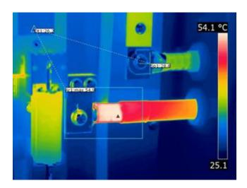
Figure 2-19: DC combiner box includes overheated interconnection with cross bar between cable and lug.
