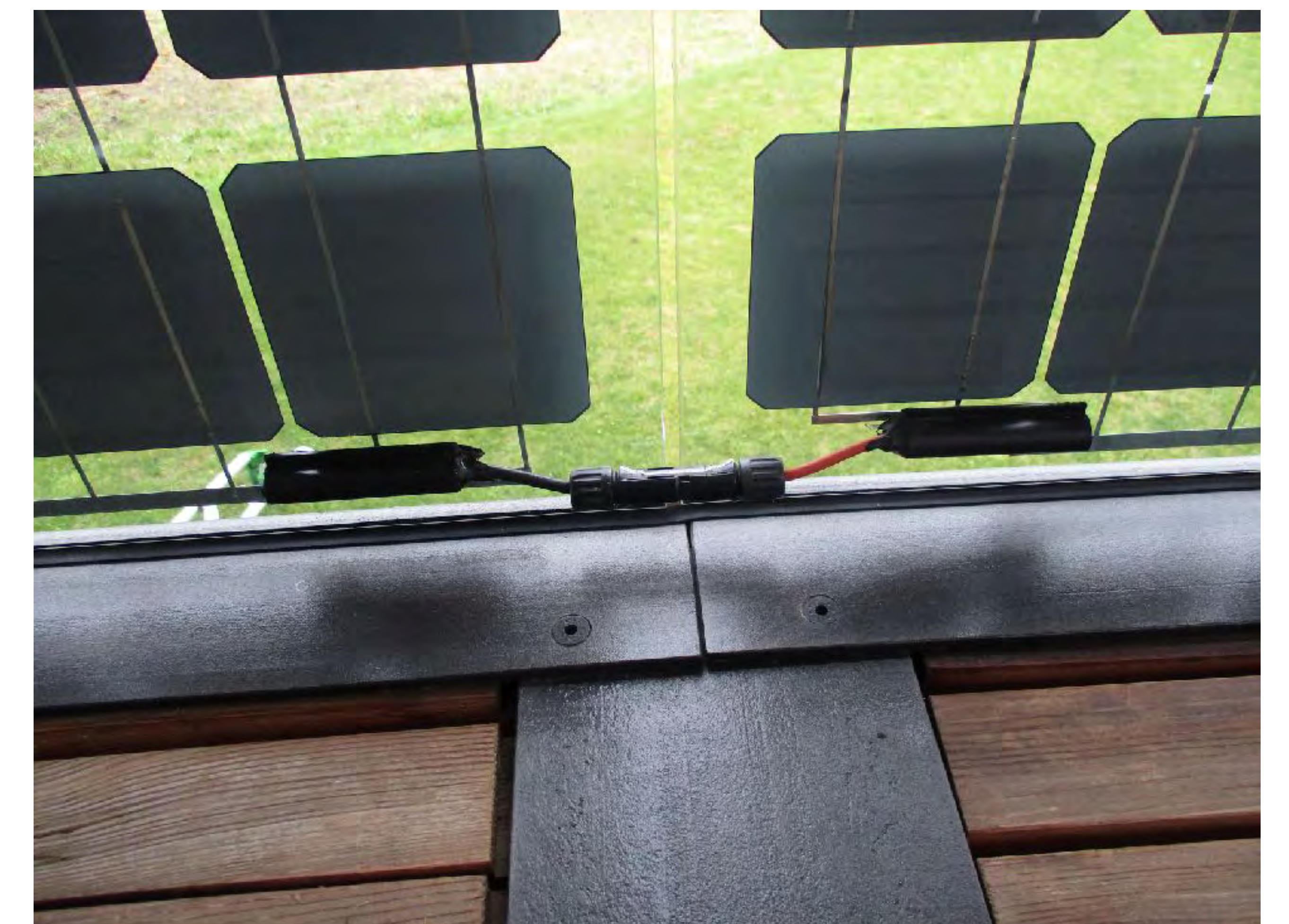
20-04. Detailed view of the junction between module cables.
