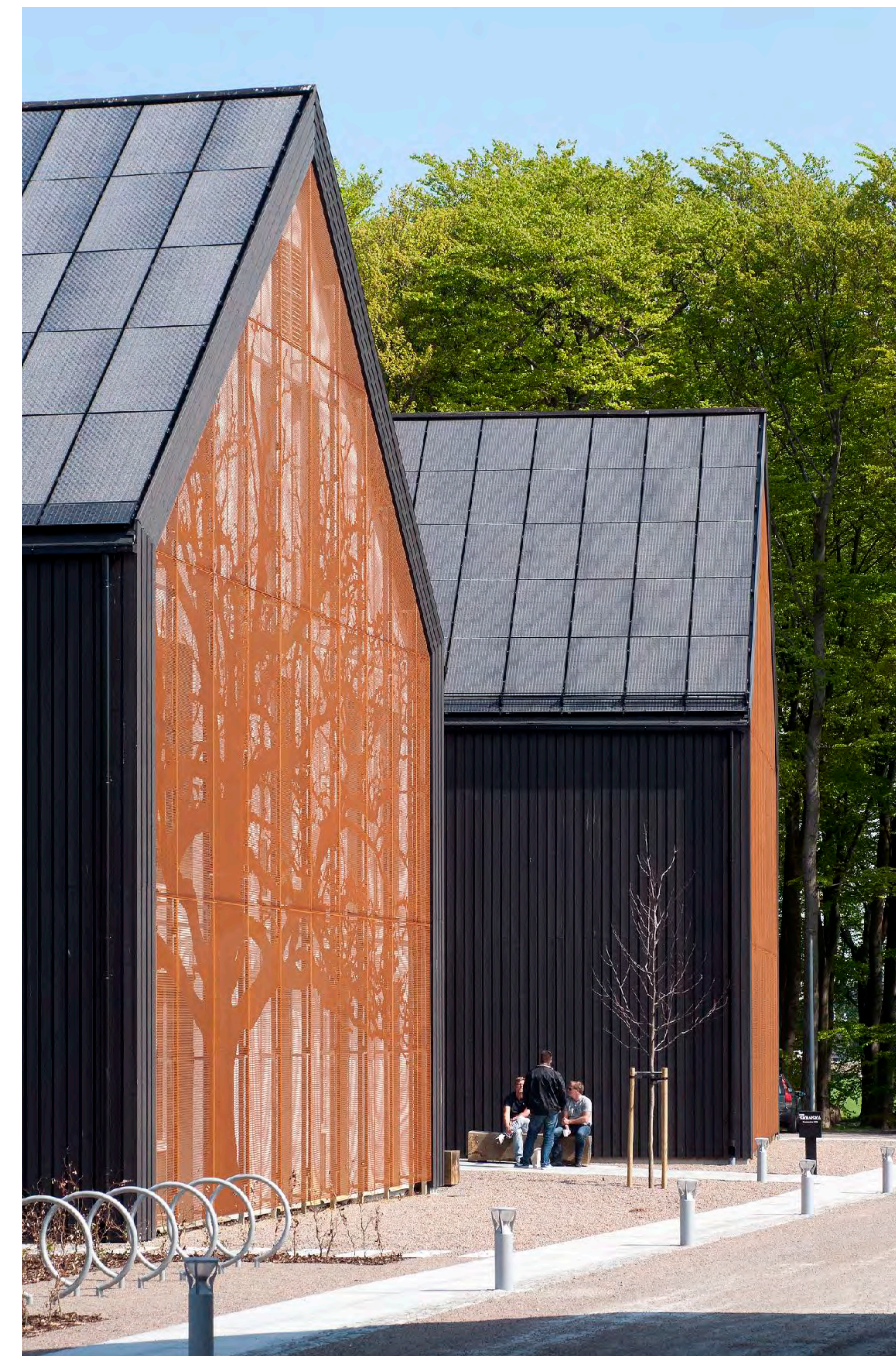
16-09. PV modules aligned with ridge and roof edge.
