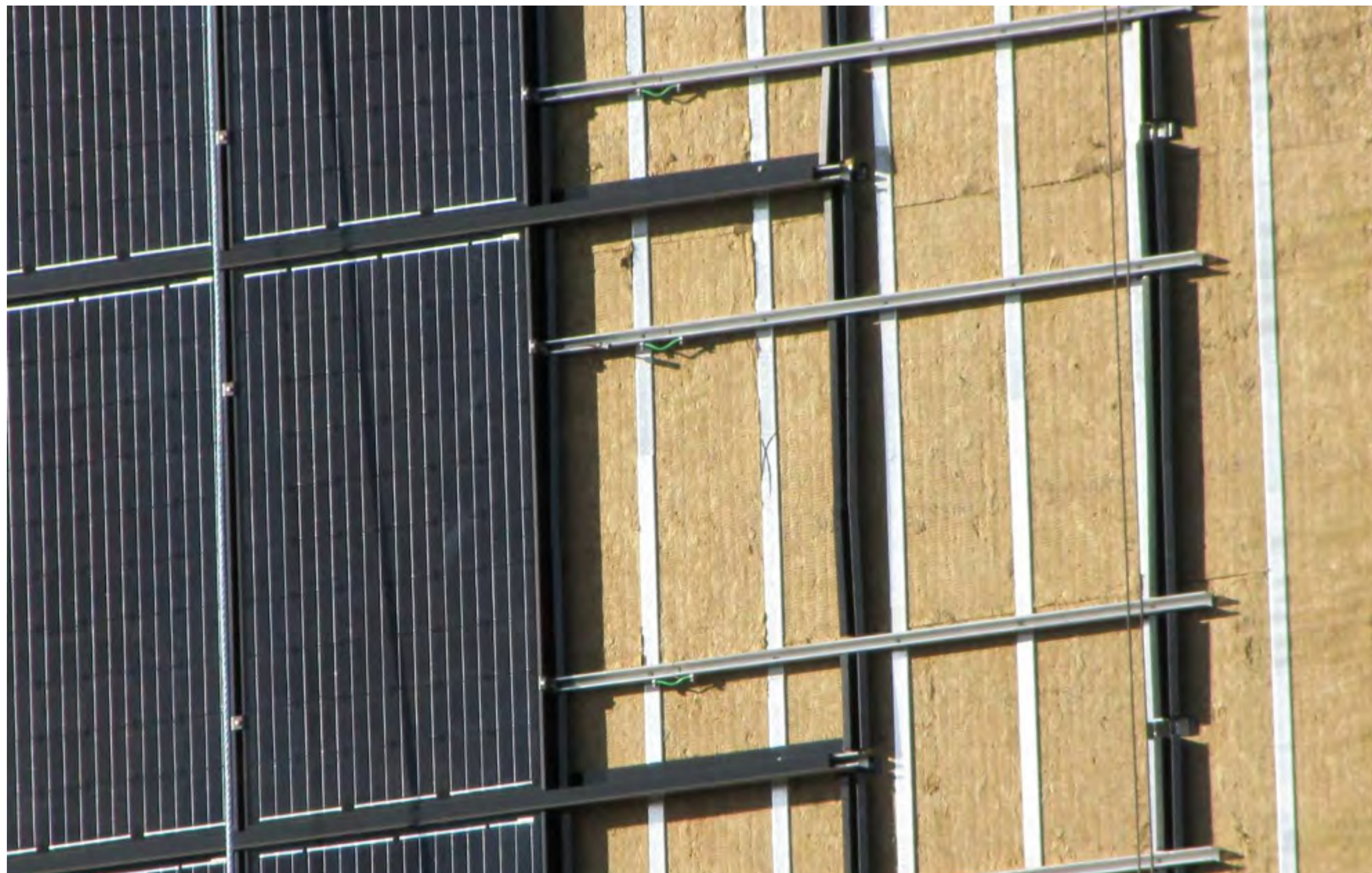
1-05. Mounted solar modules showing vertical Z-girts, insulation, horizontal Unistrut clamping rails, horizontal Unistrut sitting rail, horizontal flashing, vertical flashing and inter-strut electrical bonding.
