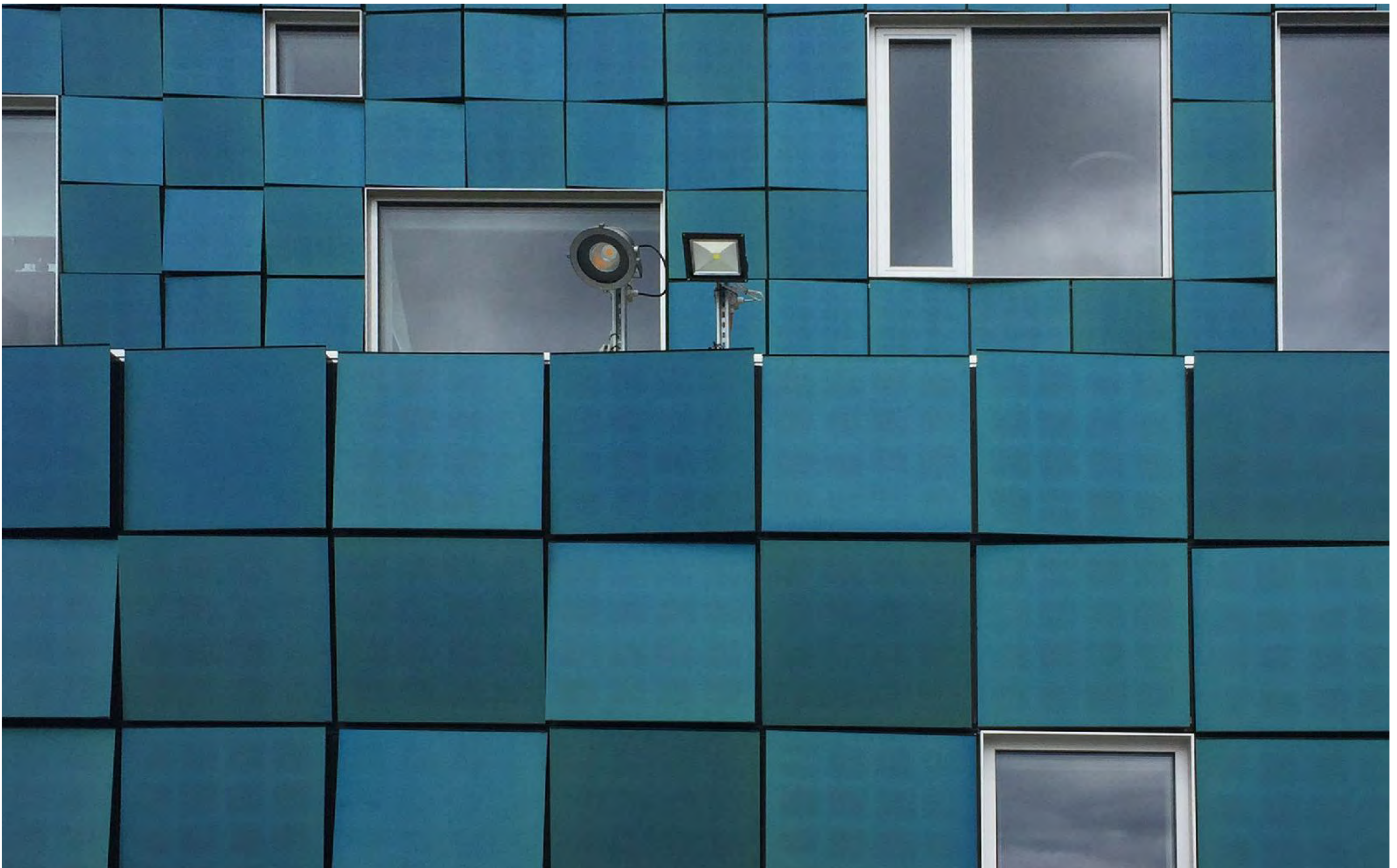
4-07. The angle of the modules within the façade creates different colours.
