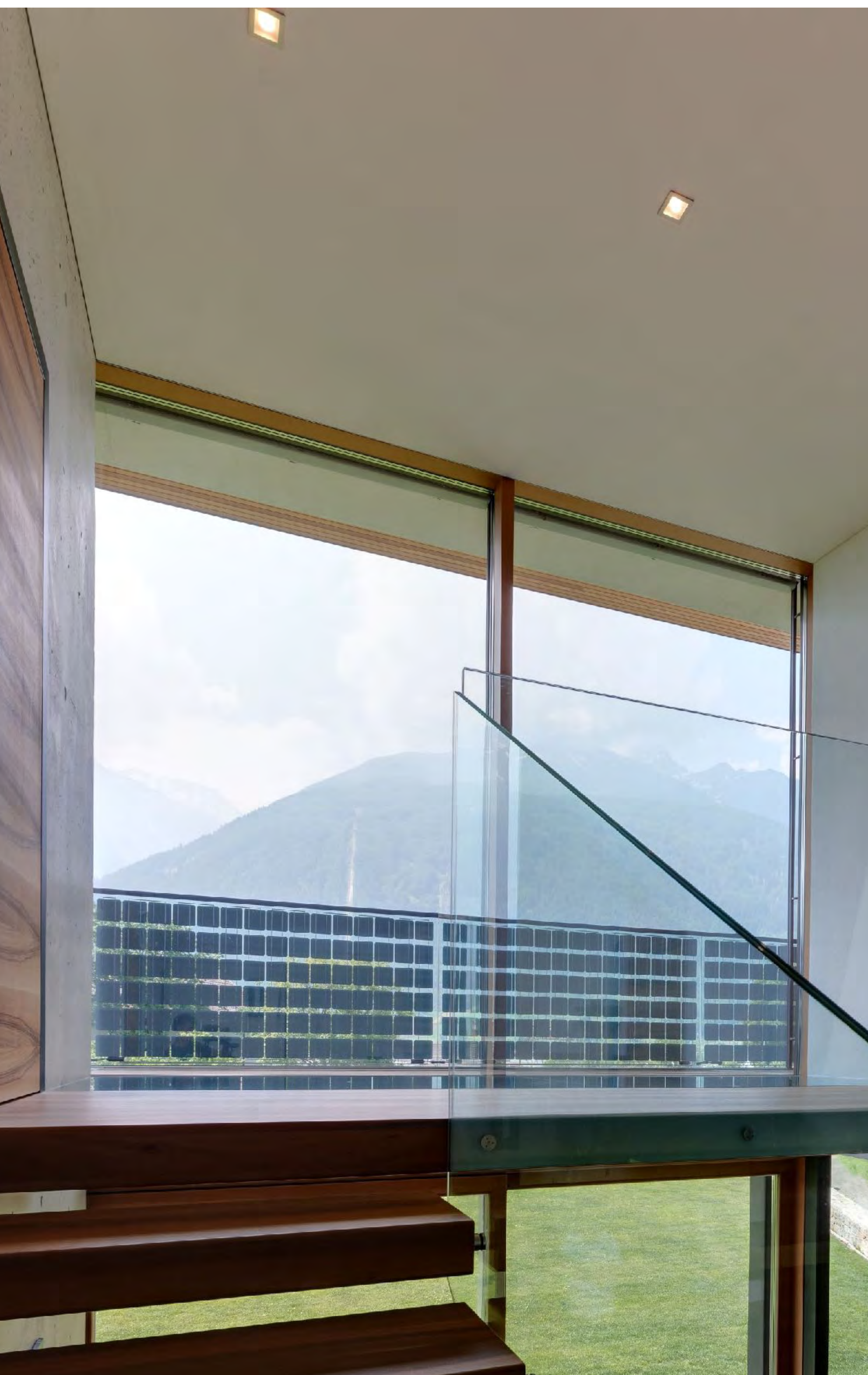
20-02. View of the photovoltaic balustrade from inside.
