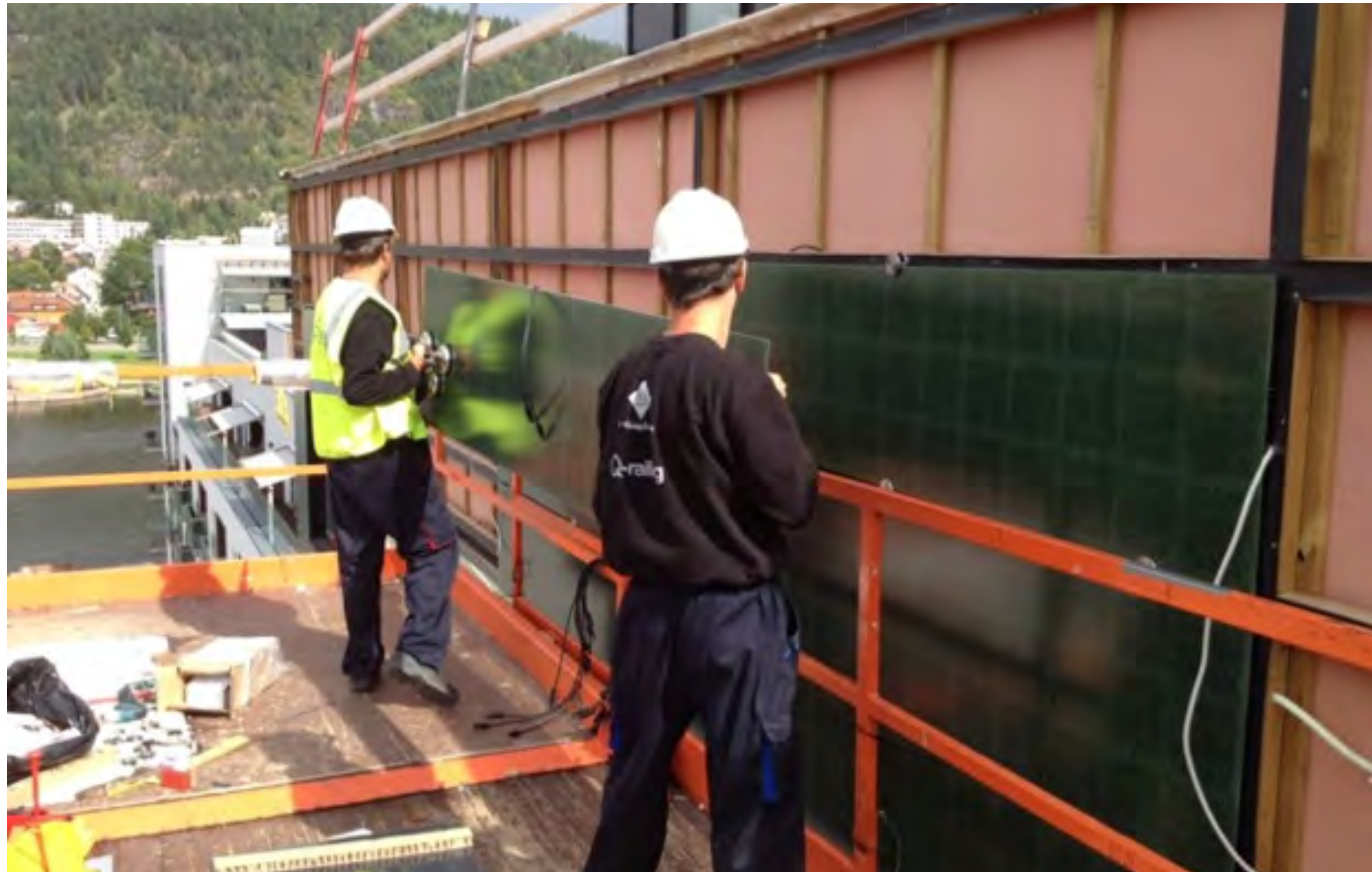
15-06. Mounting of the BIPV façade modules.
