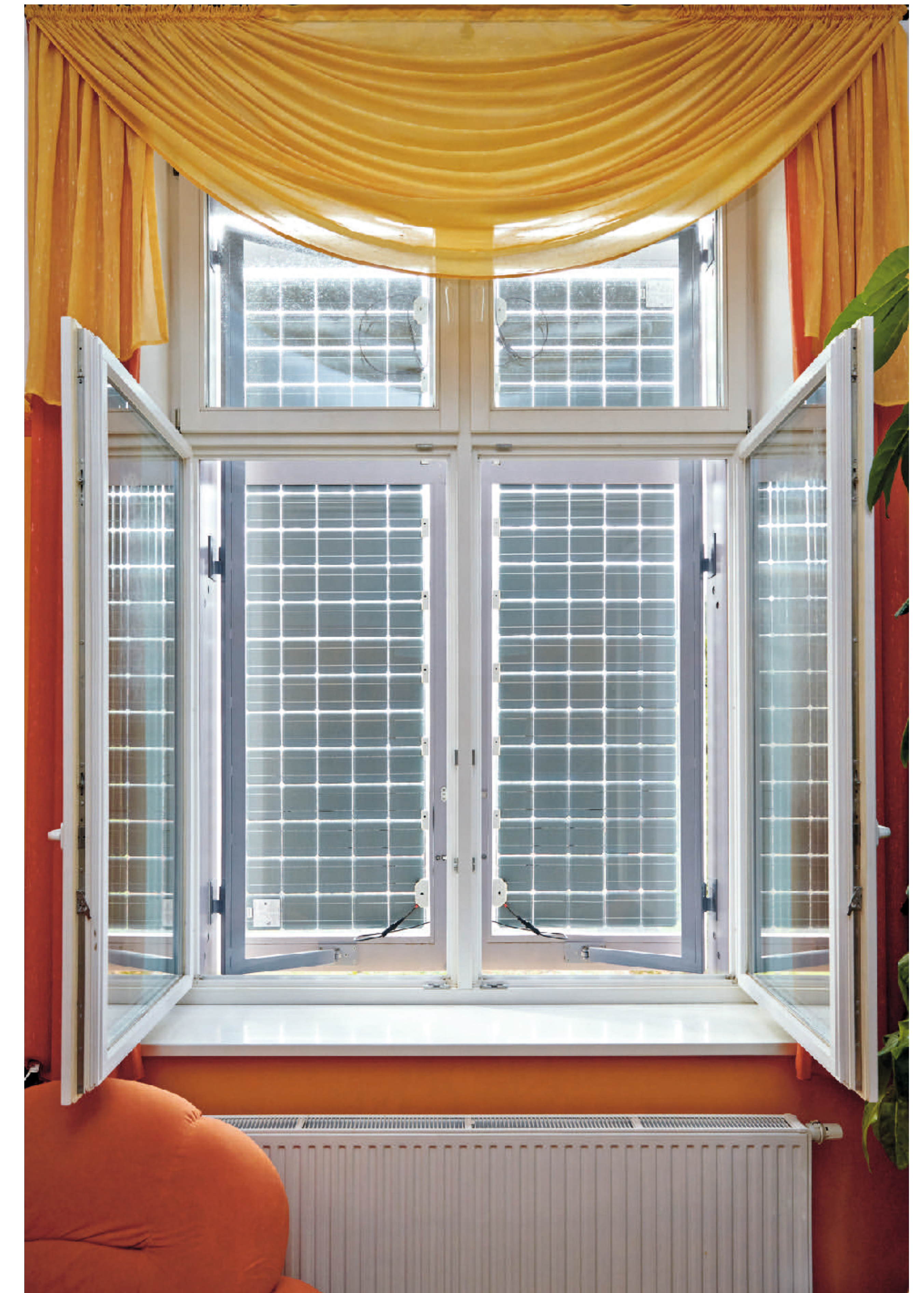
25-04. BIPV shutters in ventilation mode.
