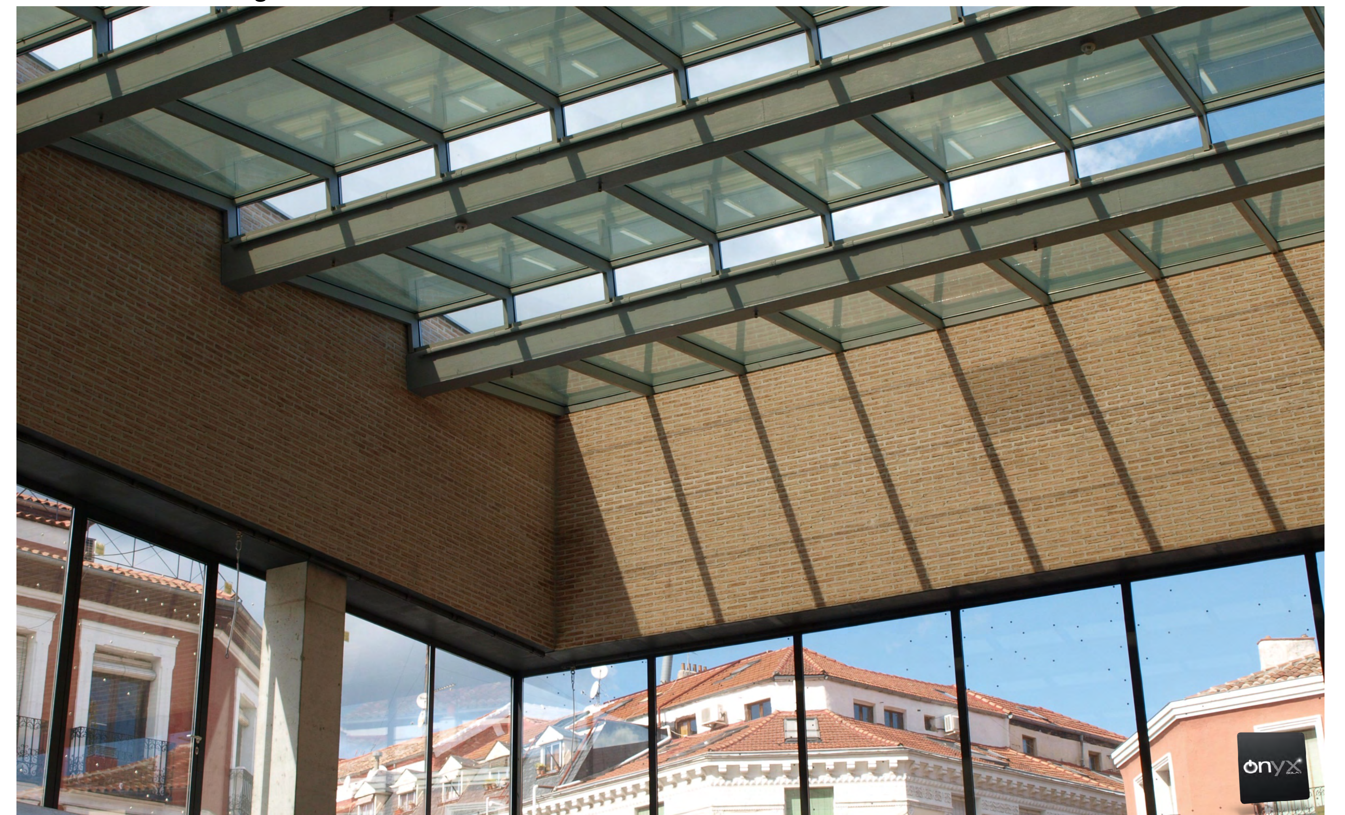
10-07. Without affecting the electricity generation, Onyx Solar Low-E photovoltaic glass reduces the infrared (90%) and ultraviolet radiation (99%) compared to with conventional laminated glass.
