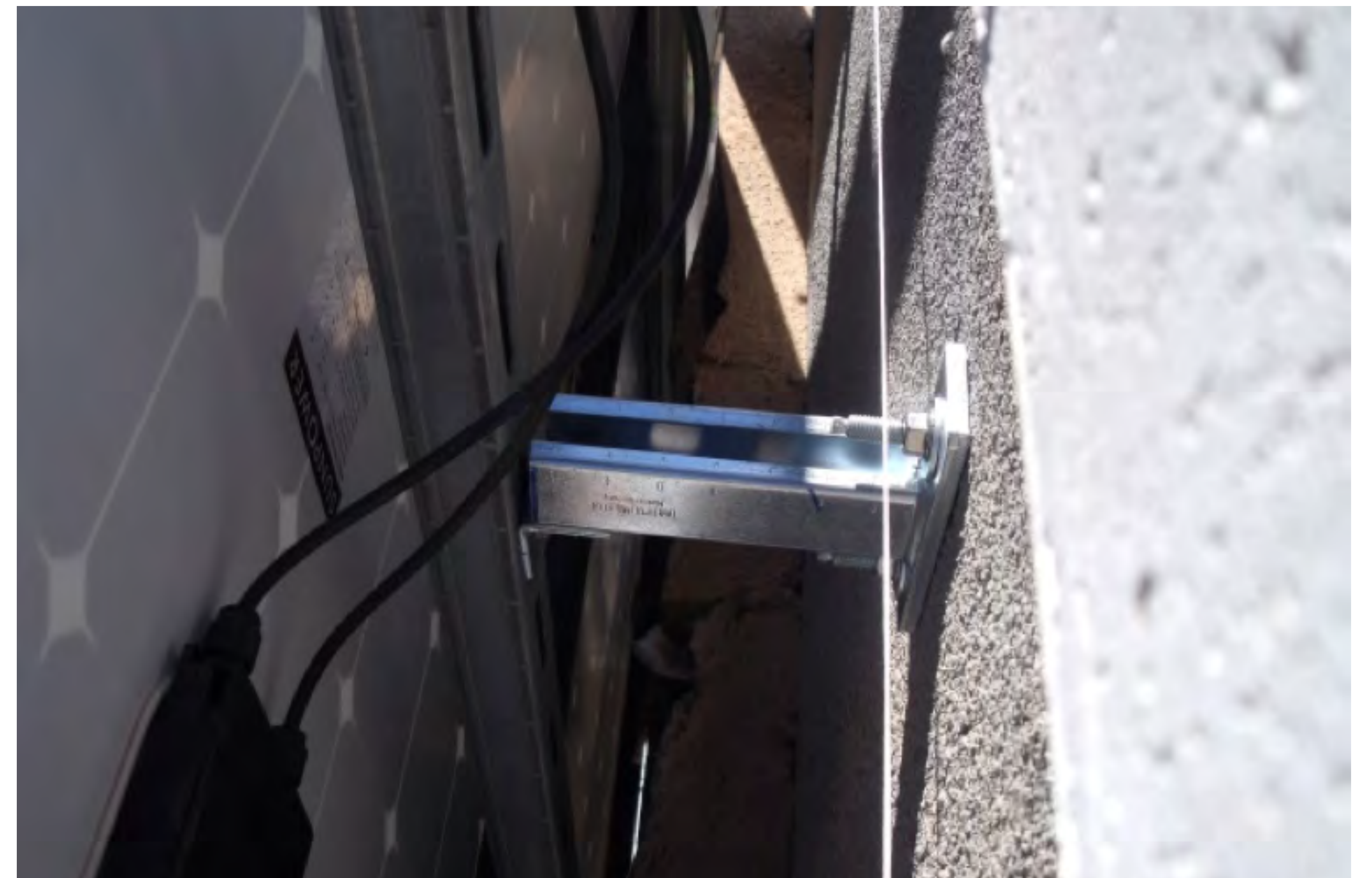
8-07. Supporting structure and fixation details behind the PV modules.
