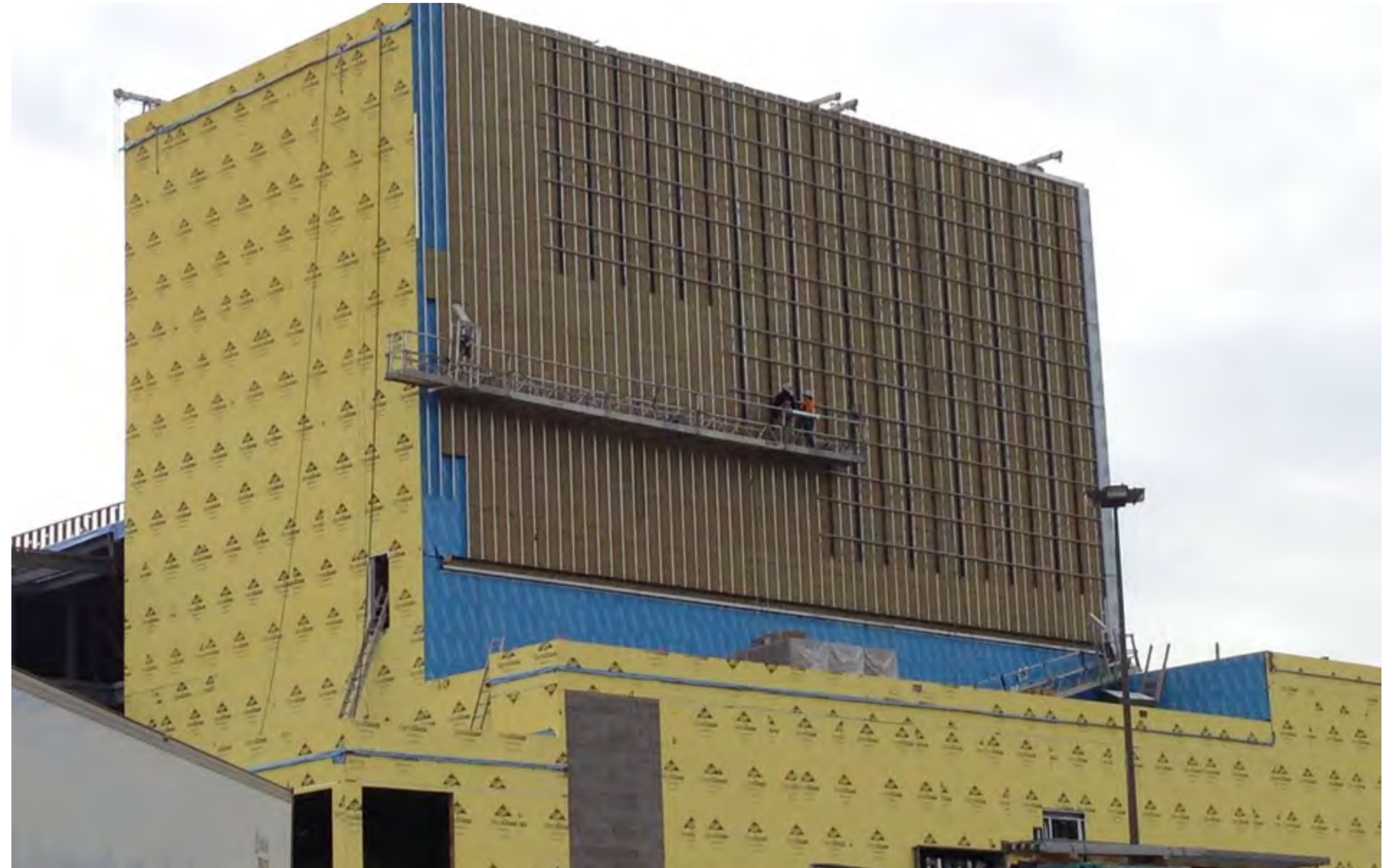
1-04. Racking system being installed on the west wall. The BIPV system serves as the building rain-screen and solar energy generator.
