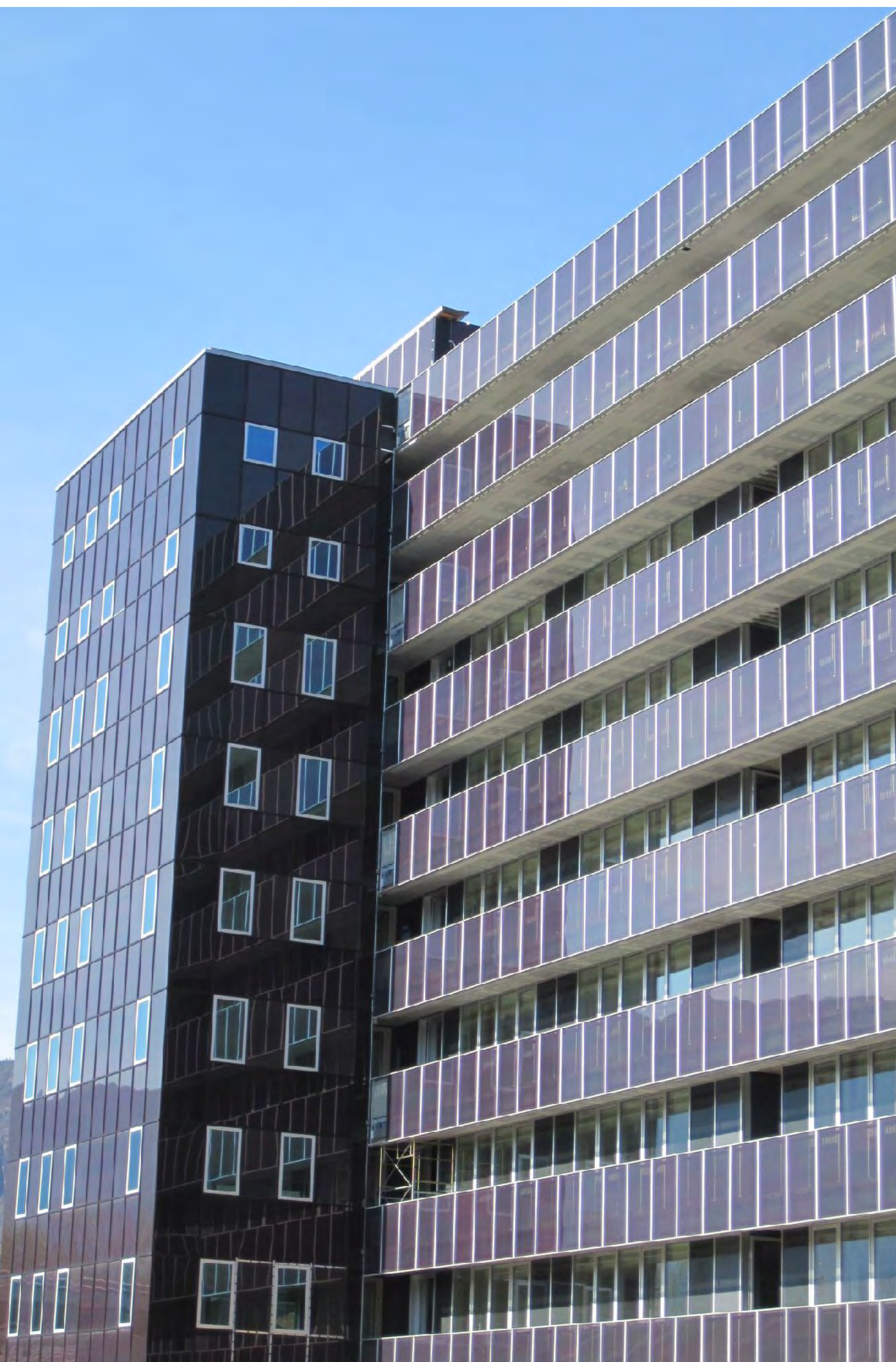
11-05. Enzian Office BIPV system: the modules replace opaque parts of the façade (horizontal bands below windows) and semi-transparent sections (horizontally between windows).
