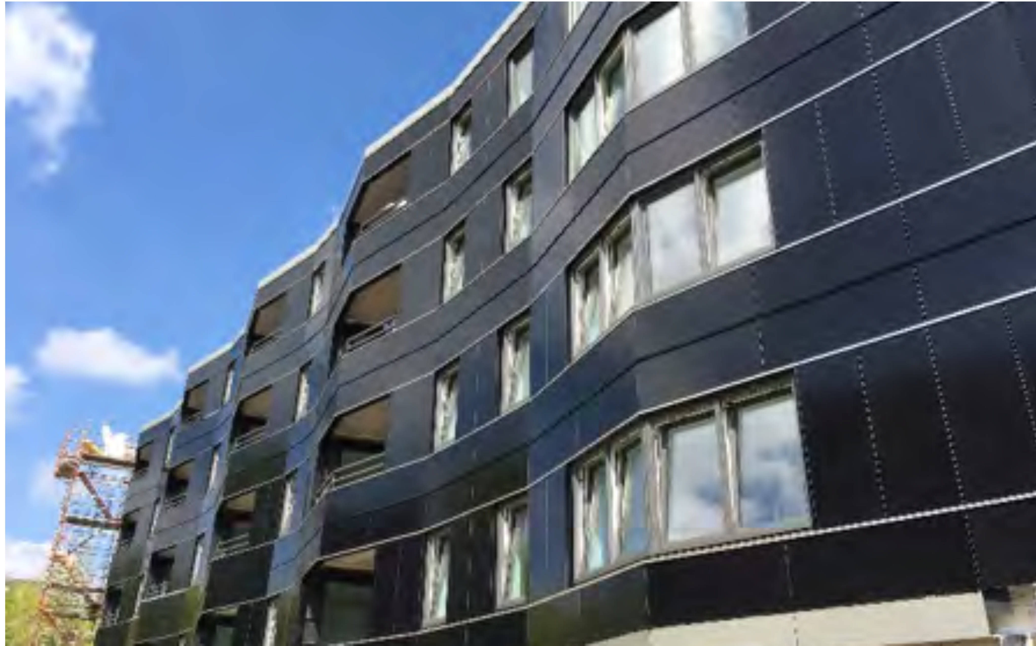
21-04. Because of standard dimensions, the PV modules are installed in a zigzag shape.
