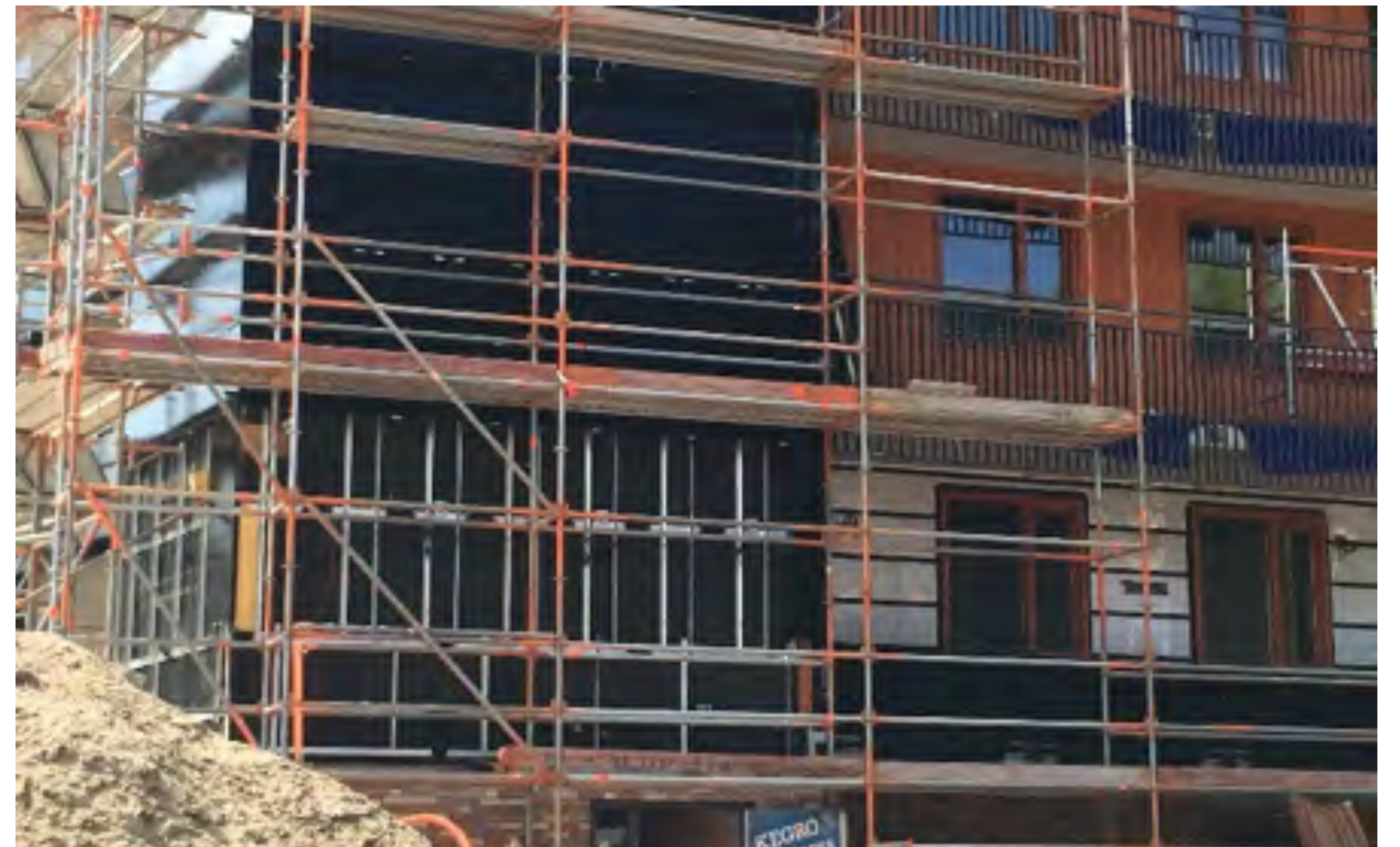
21-07. The outer layer of the traditional cavity wall is replaced by BIPV.
