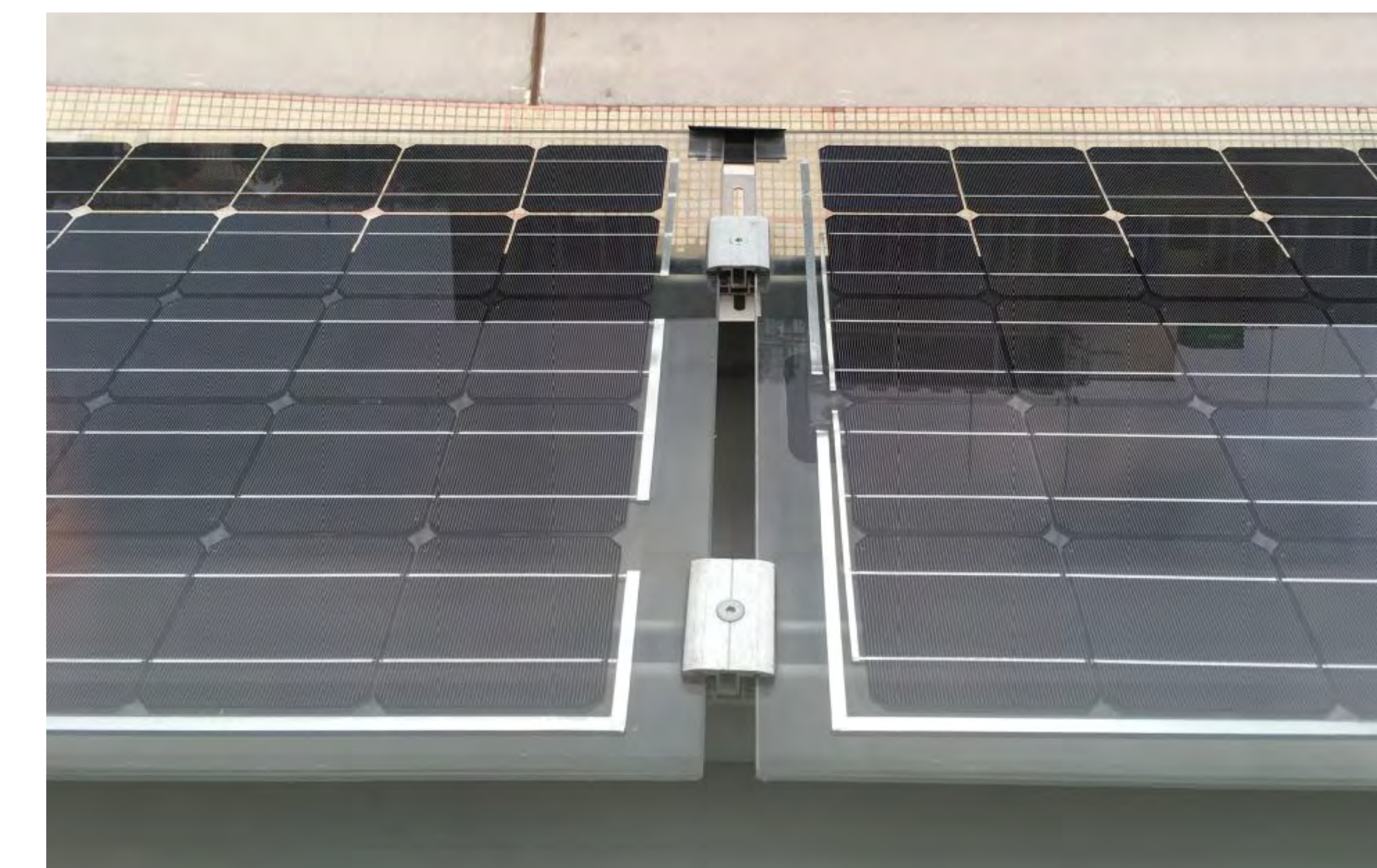
7-08 Detail of the fixation.
