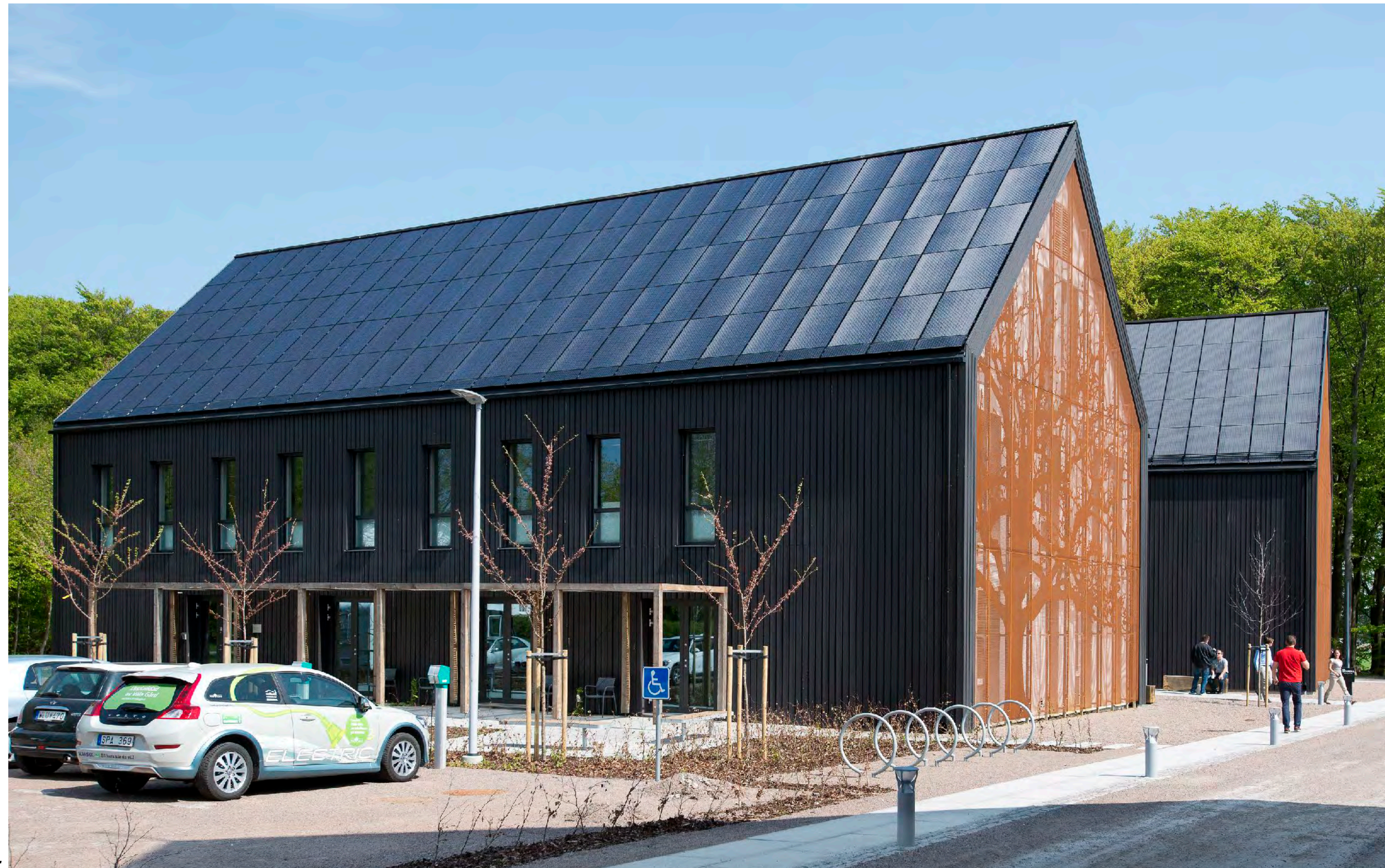
16-03. South façade and BIPV roof.
