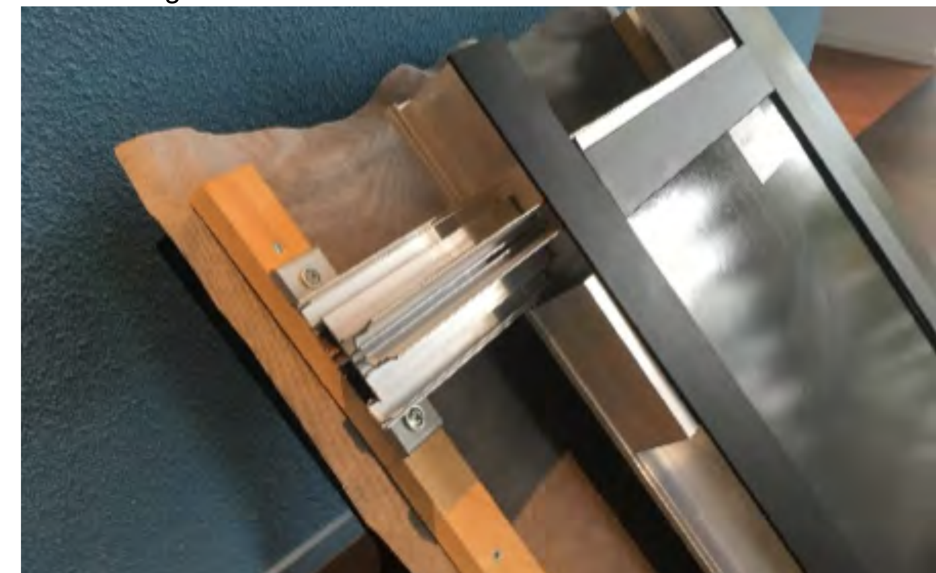
19-05 Basic detail of the roof integration.
