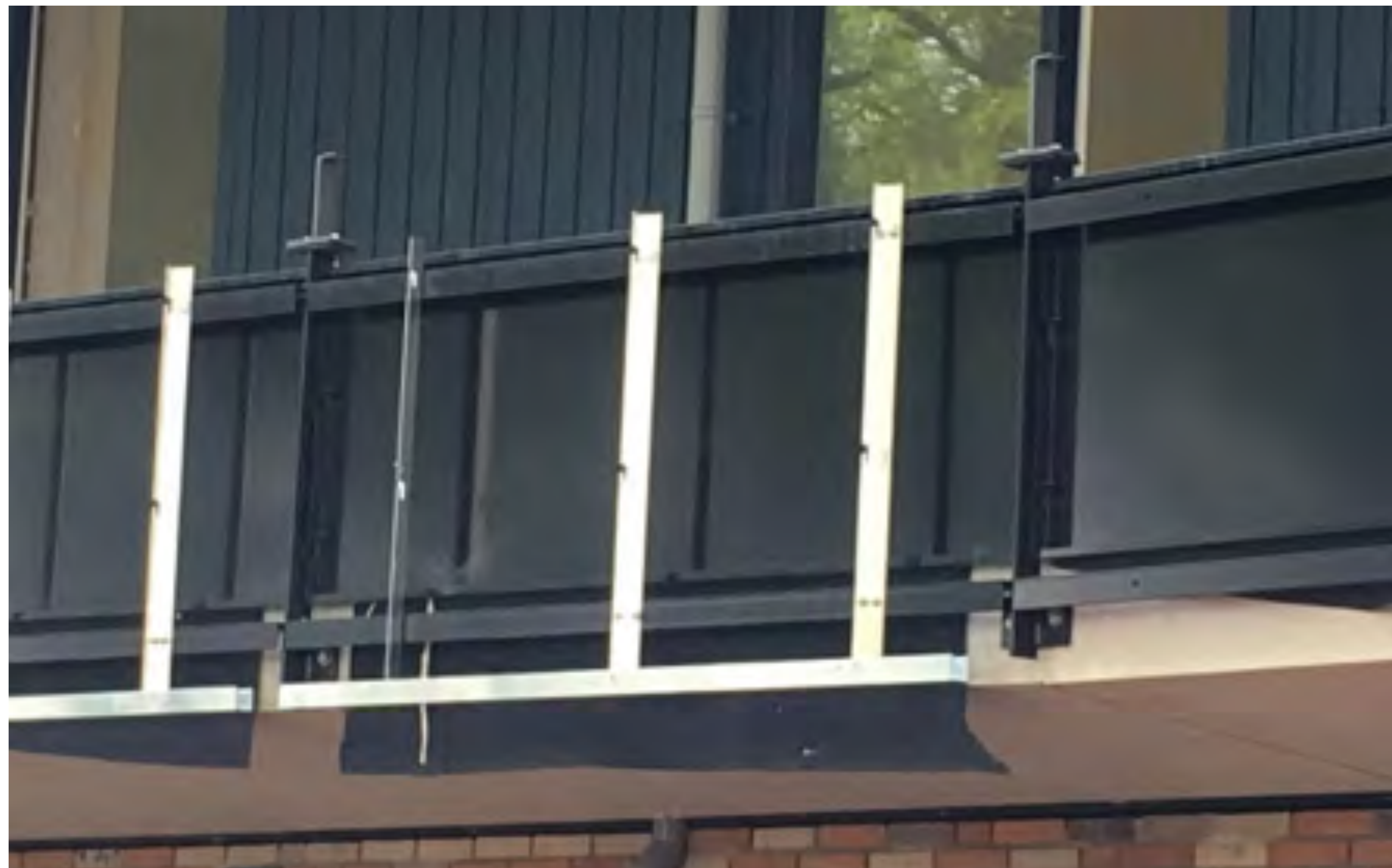
21-06. The modules are mounted on an aluminum support structure.
