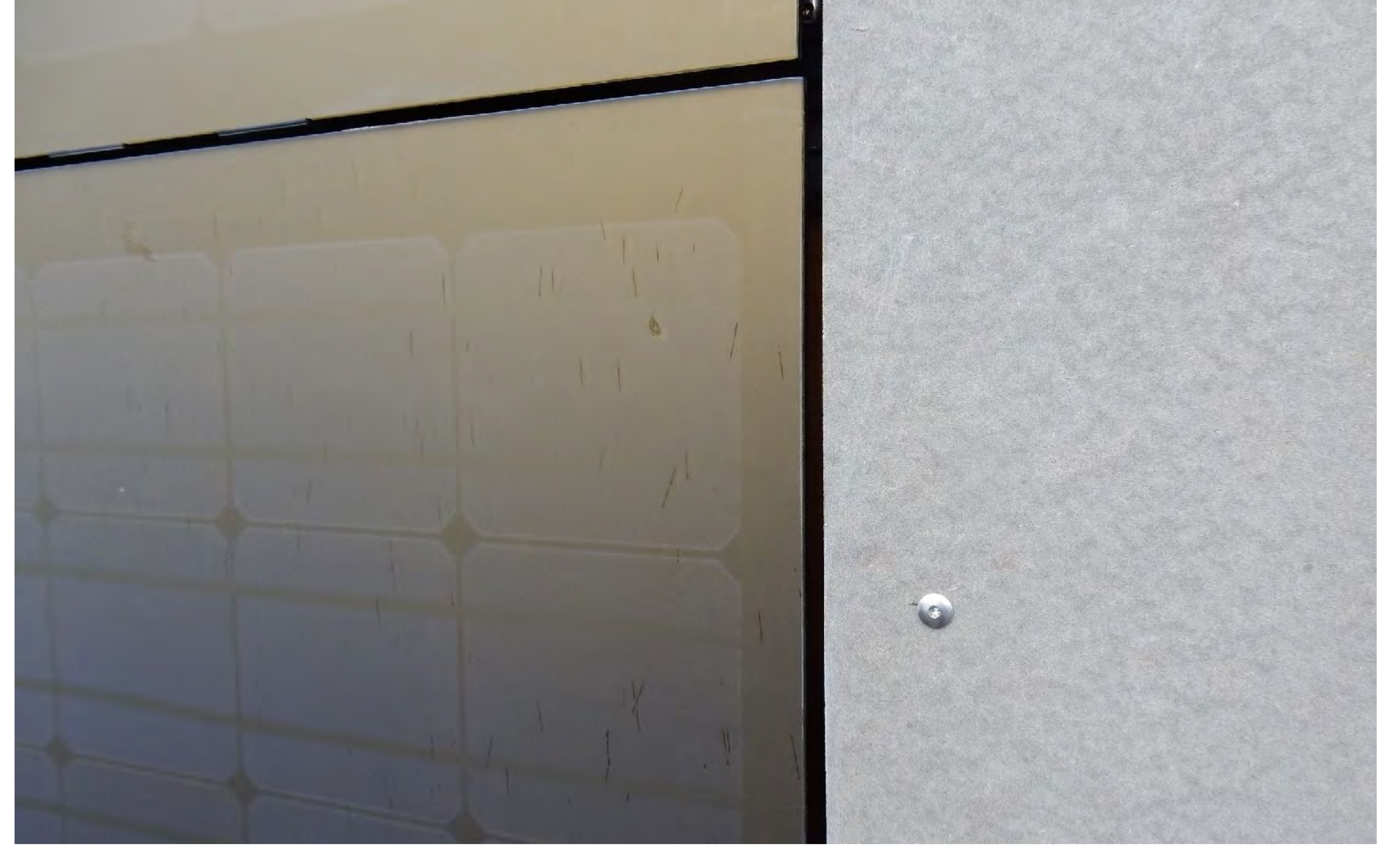
17-08. Detail of the façade PV cladding with hidden solar cells.
