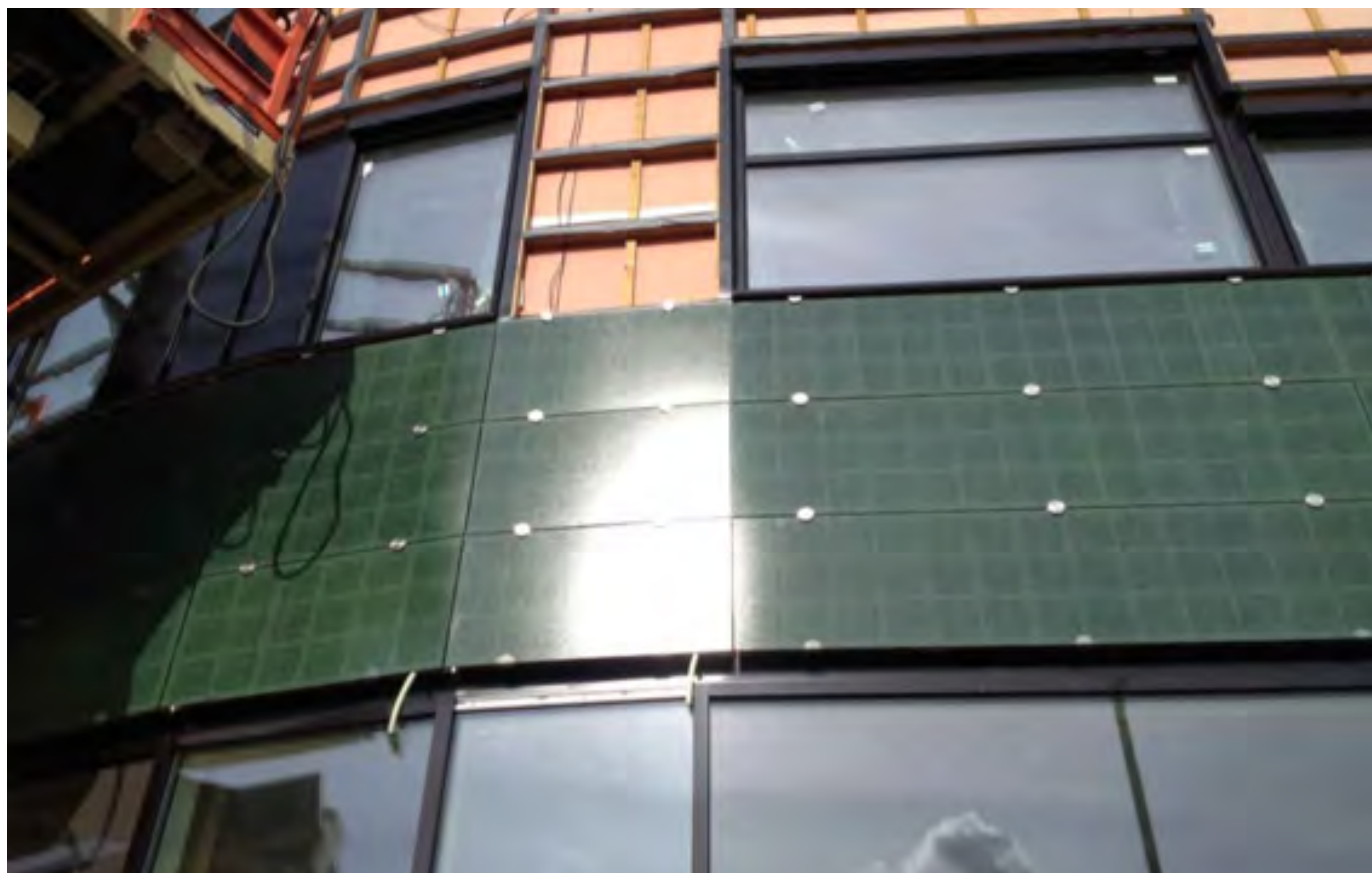
15-08. Mounting BIPV modules on a curved section.
