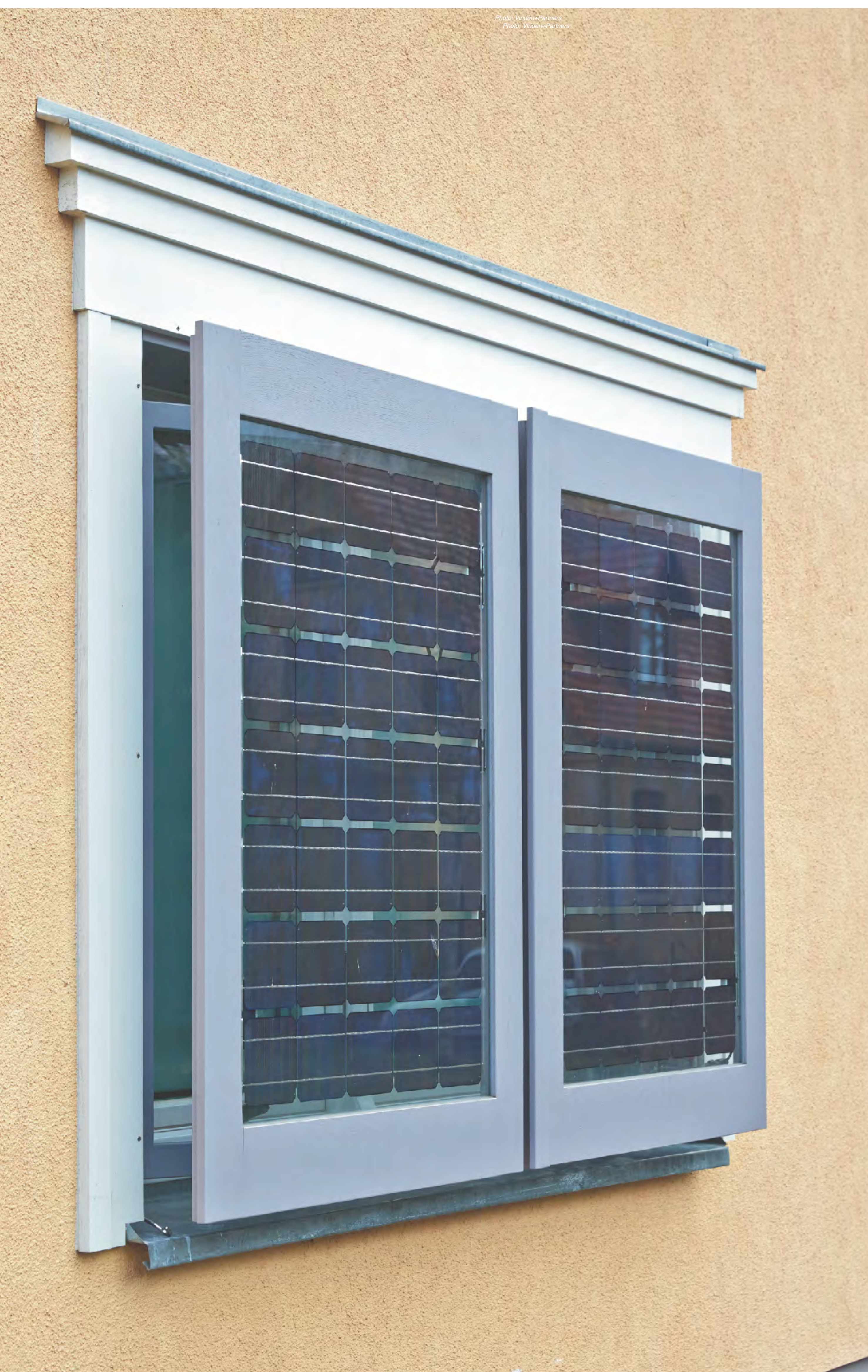
25-06. BIPV shutters in ventilation mode.
