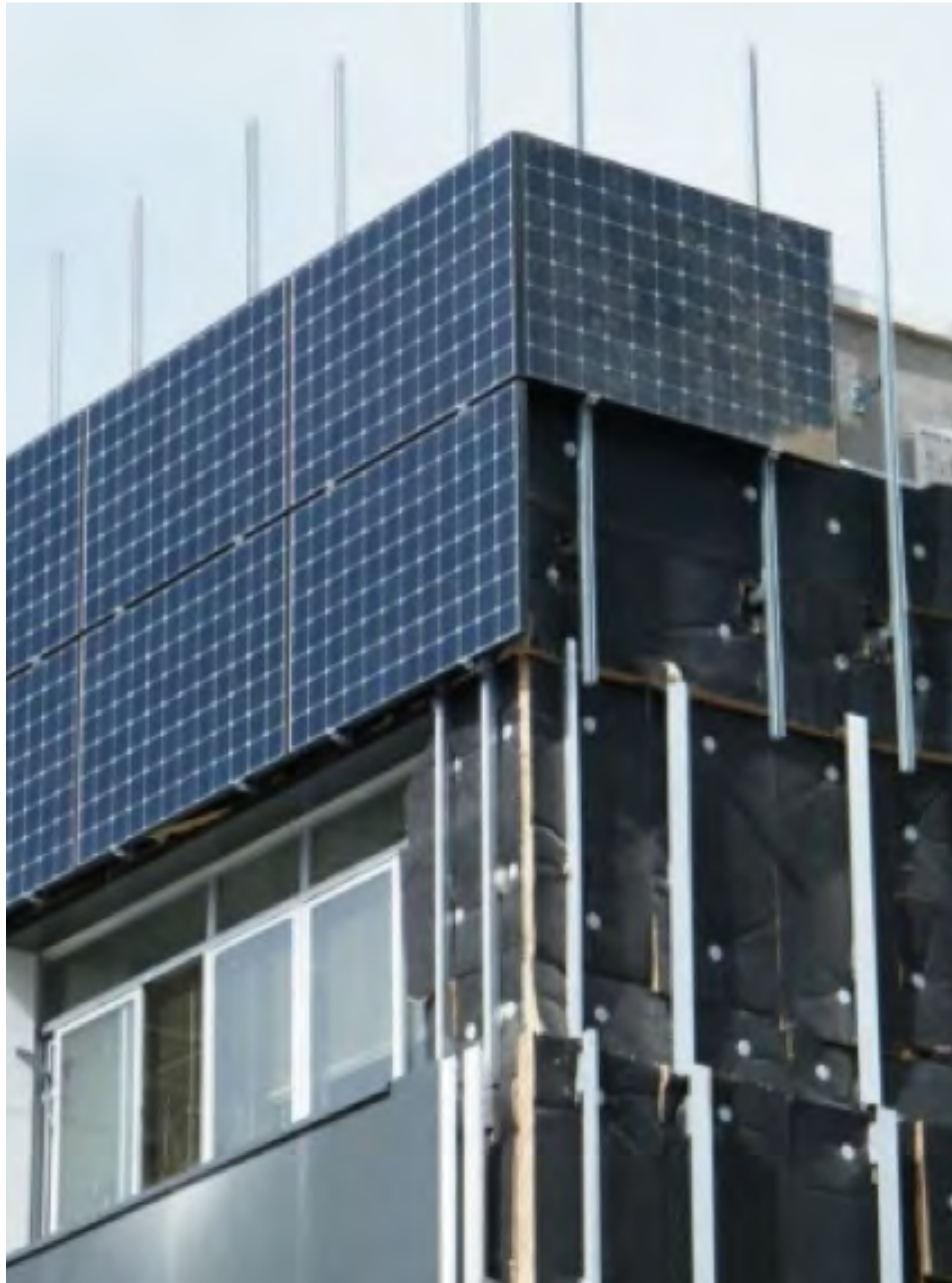
8-06. Renovation work details: mounting the PV modules.
