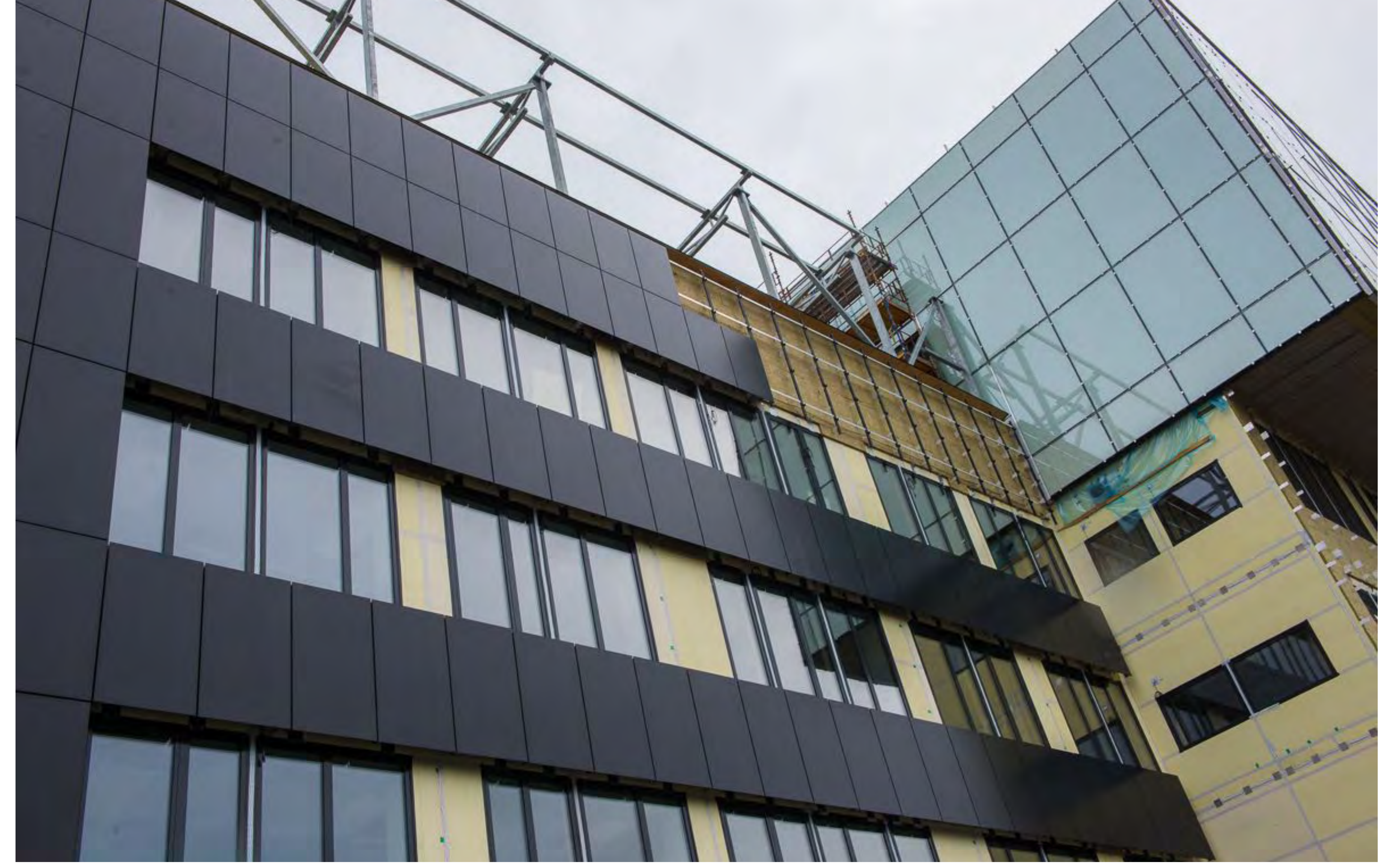
3-07. Mounting of the BIPV façade modules.
