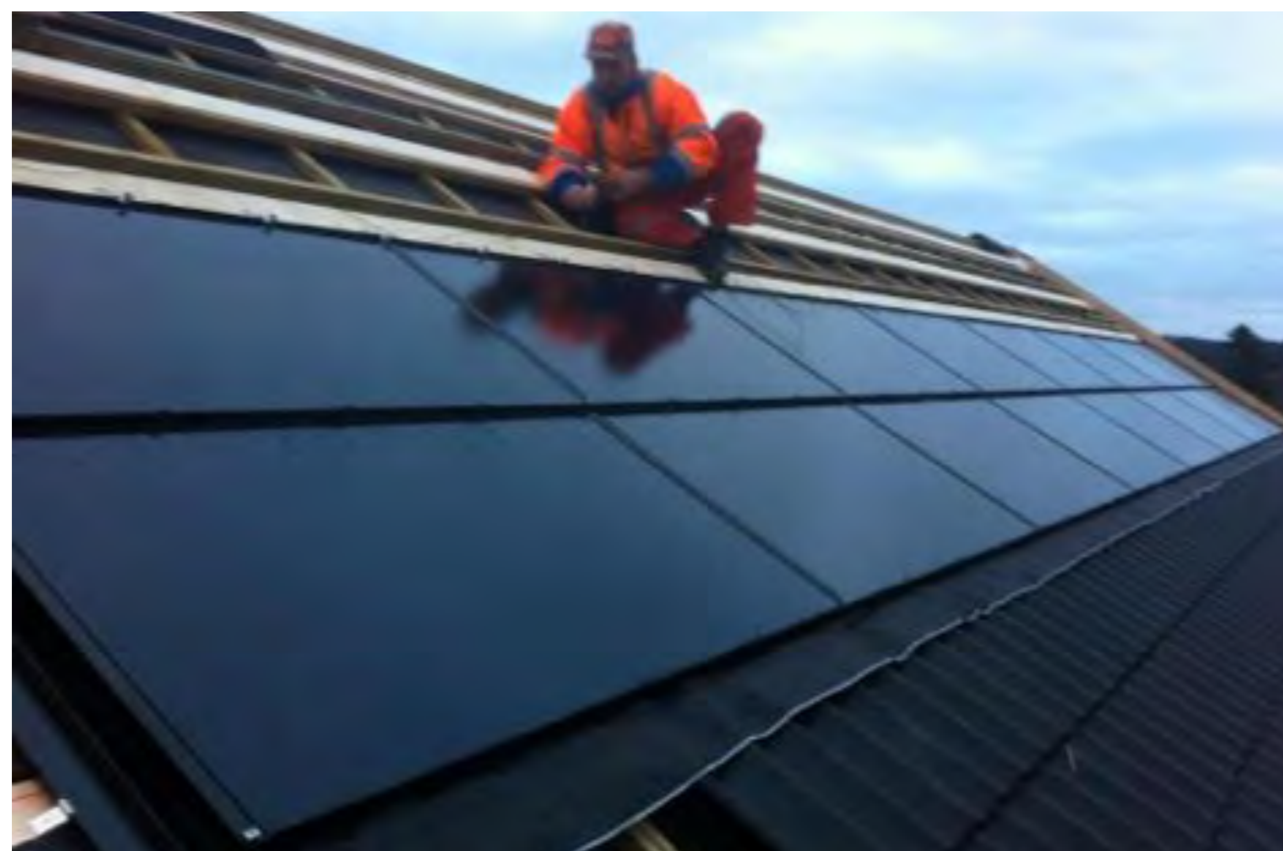
22-04. Mounting of the BIPV modules.
