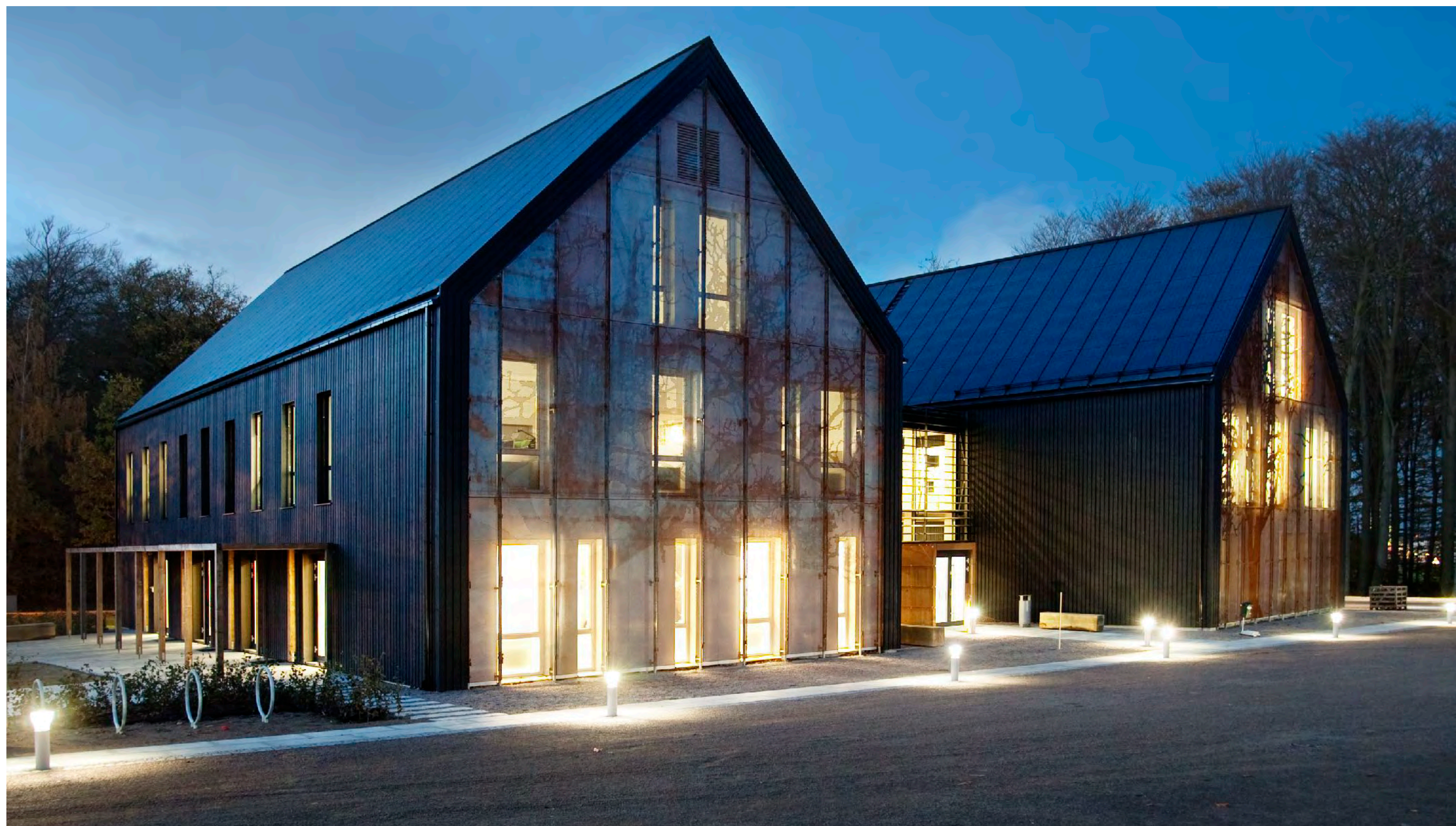
16-08. BIPV roofs for a zero-energy office.
