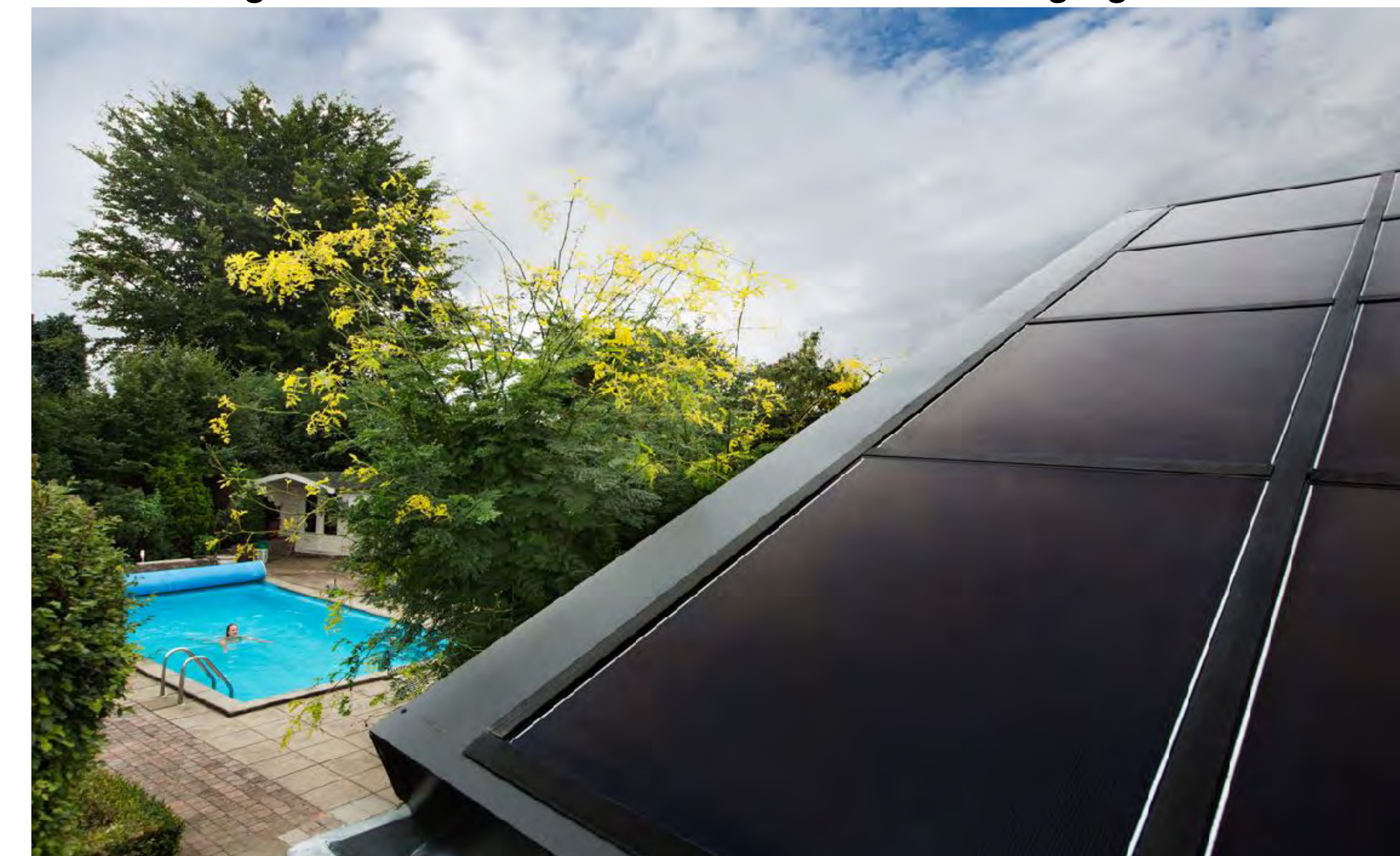
19-08 Design solution connection BIPV and eaves (top-view).
