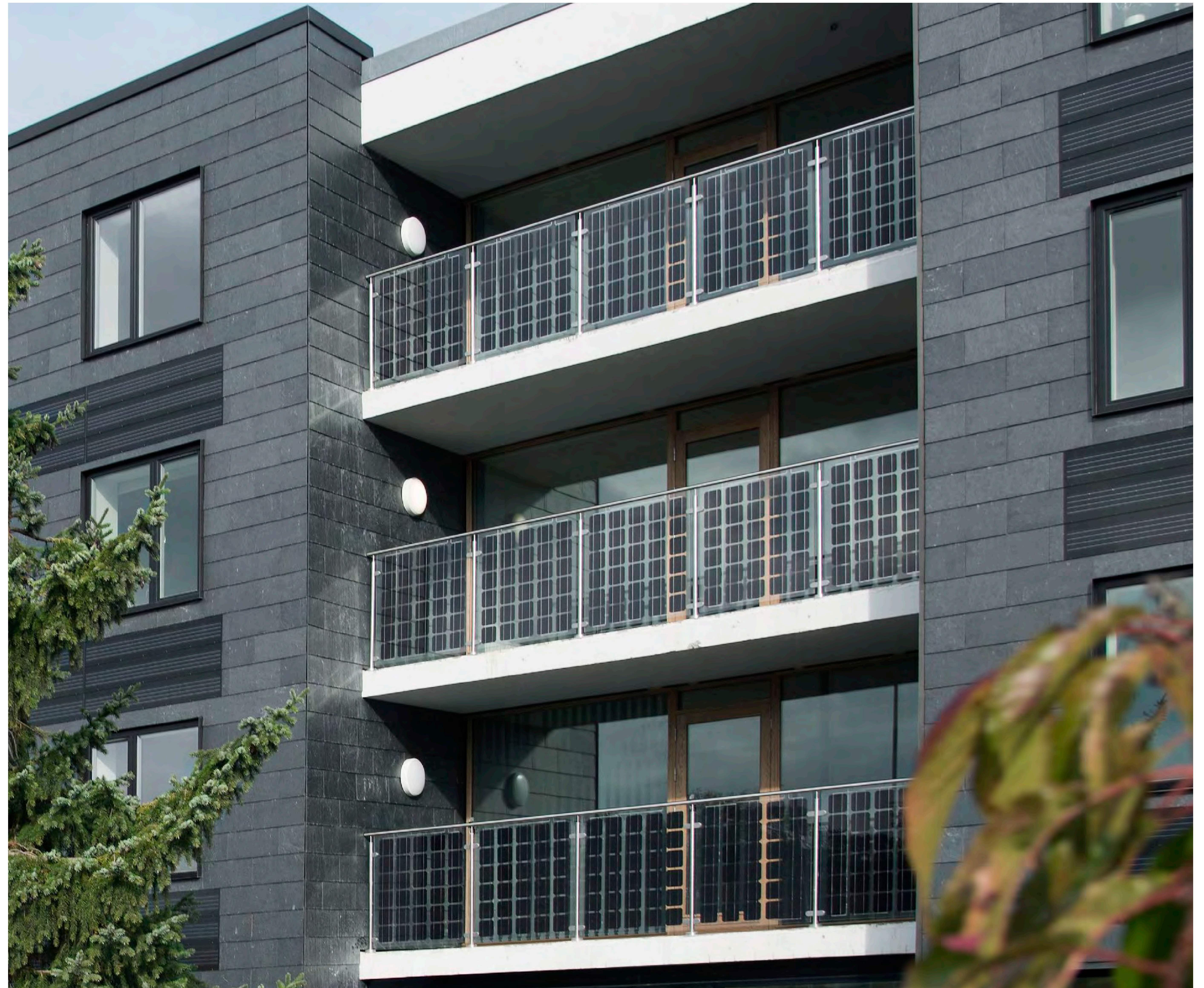
18-09. Semi-transparent modules in the balustrades.
