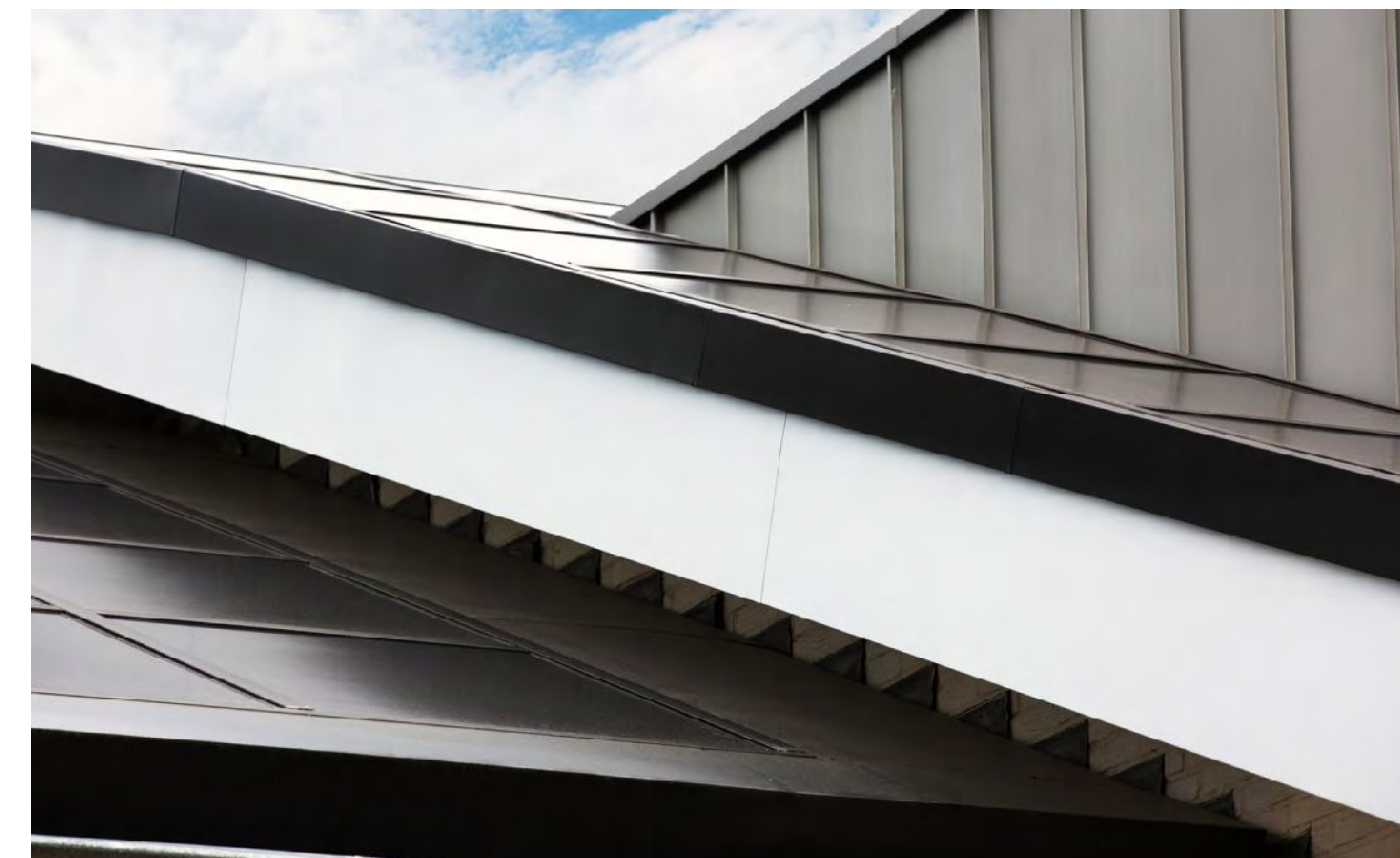
19-07 Design solution connection BIPV and overhanging eaves.
