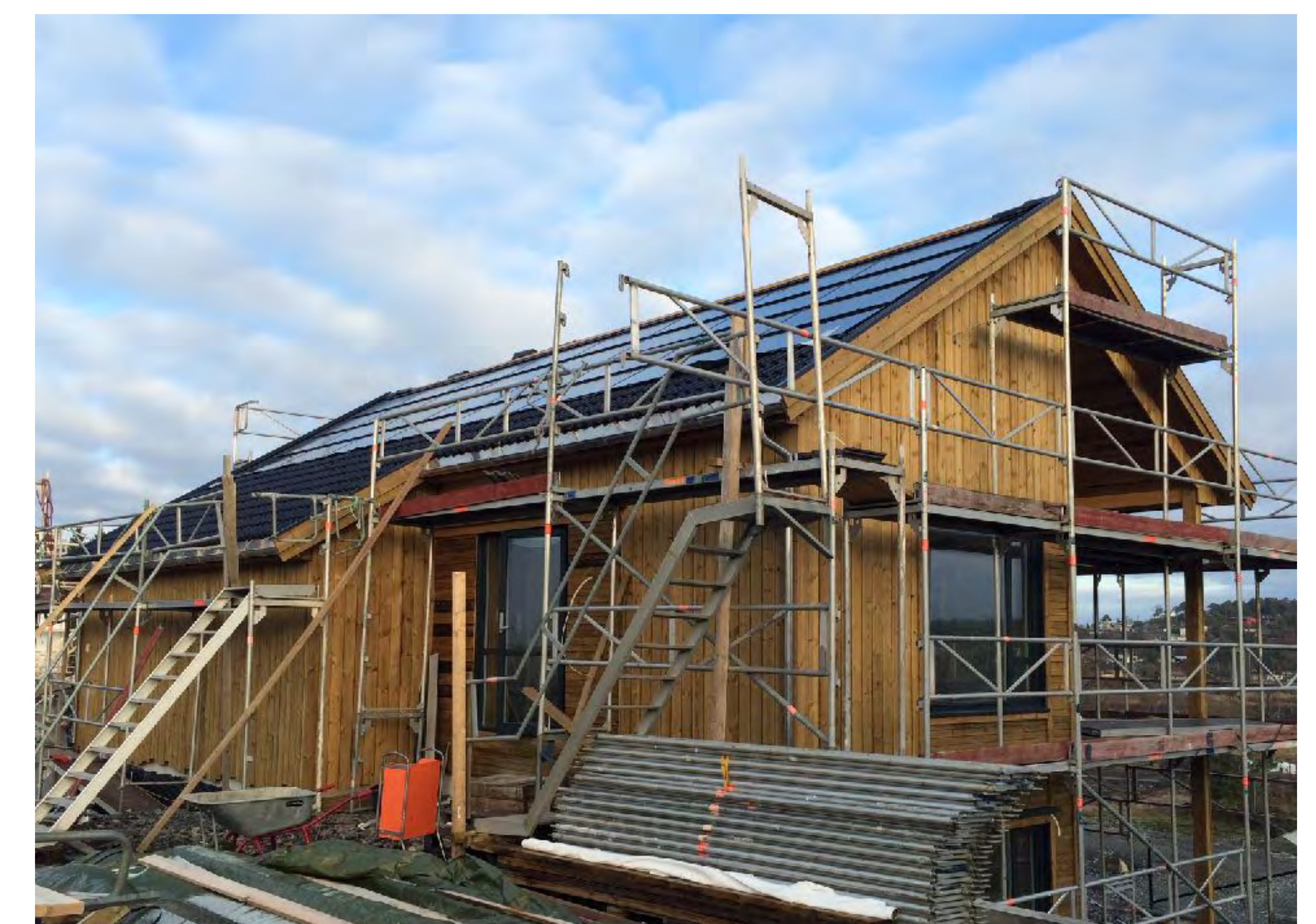
22-03. Building site after BIPV installation.
