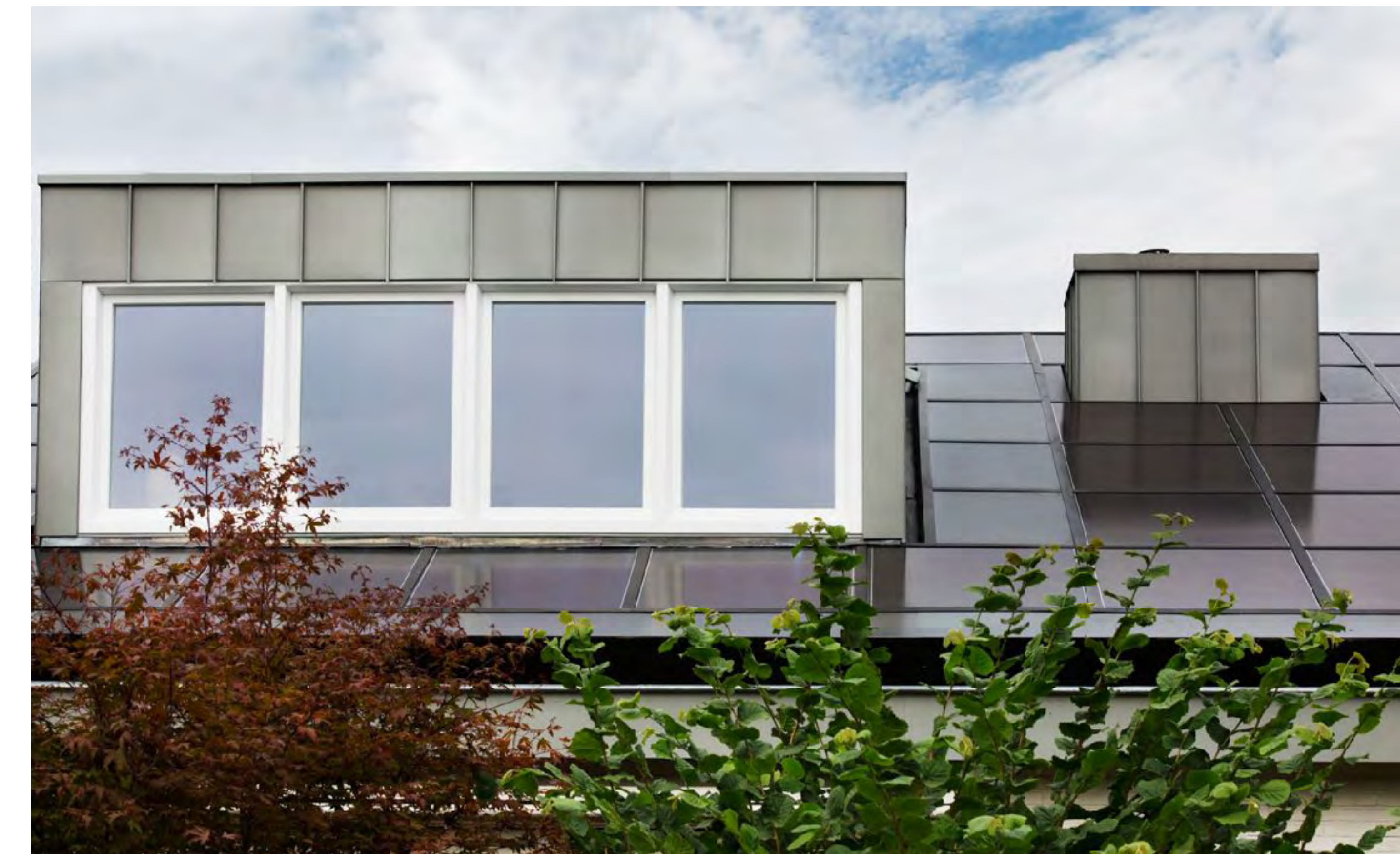
19-04 Design solution connection BIPV and dormer.
