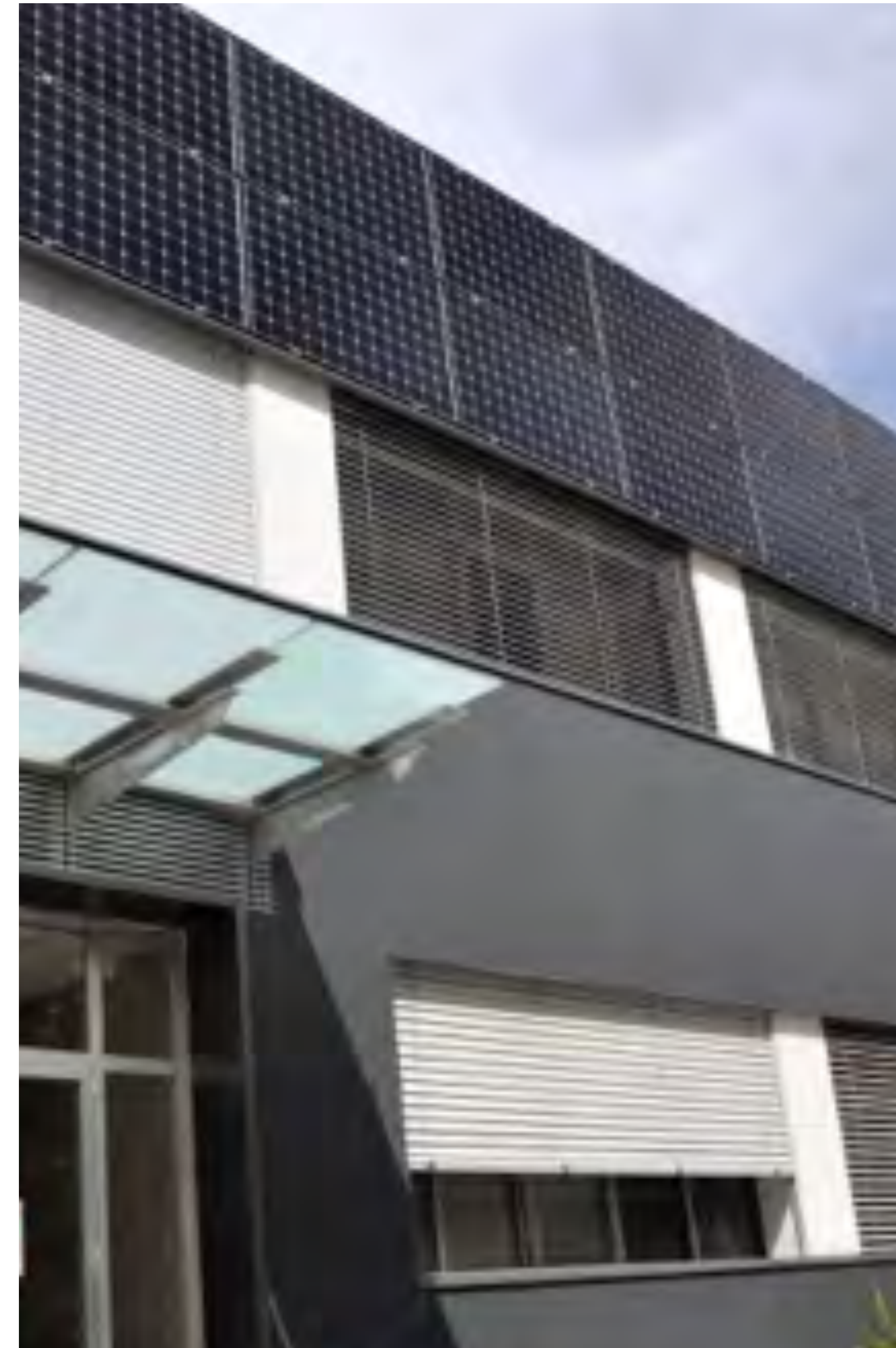
8-03. CIEMAT office renovation with BIPV cladding.
