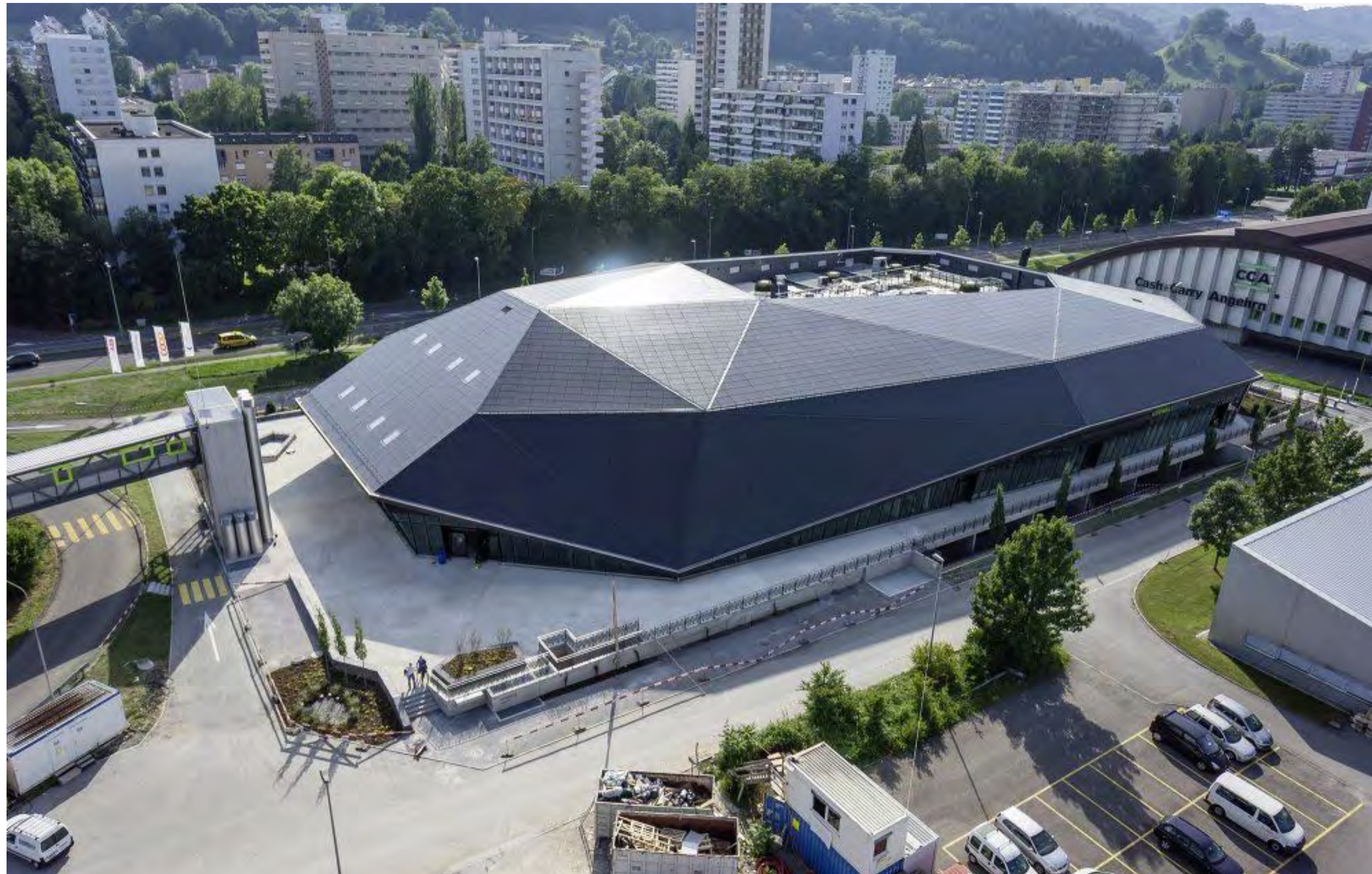
5-07. The BIPV roof system (5,300 m 2 ), generates around 540,000 kWh of electricity per year.
