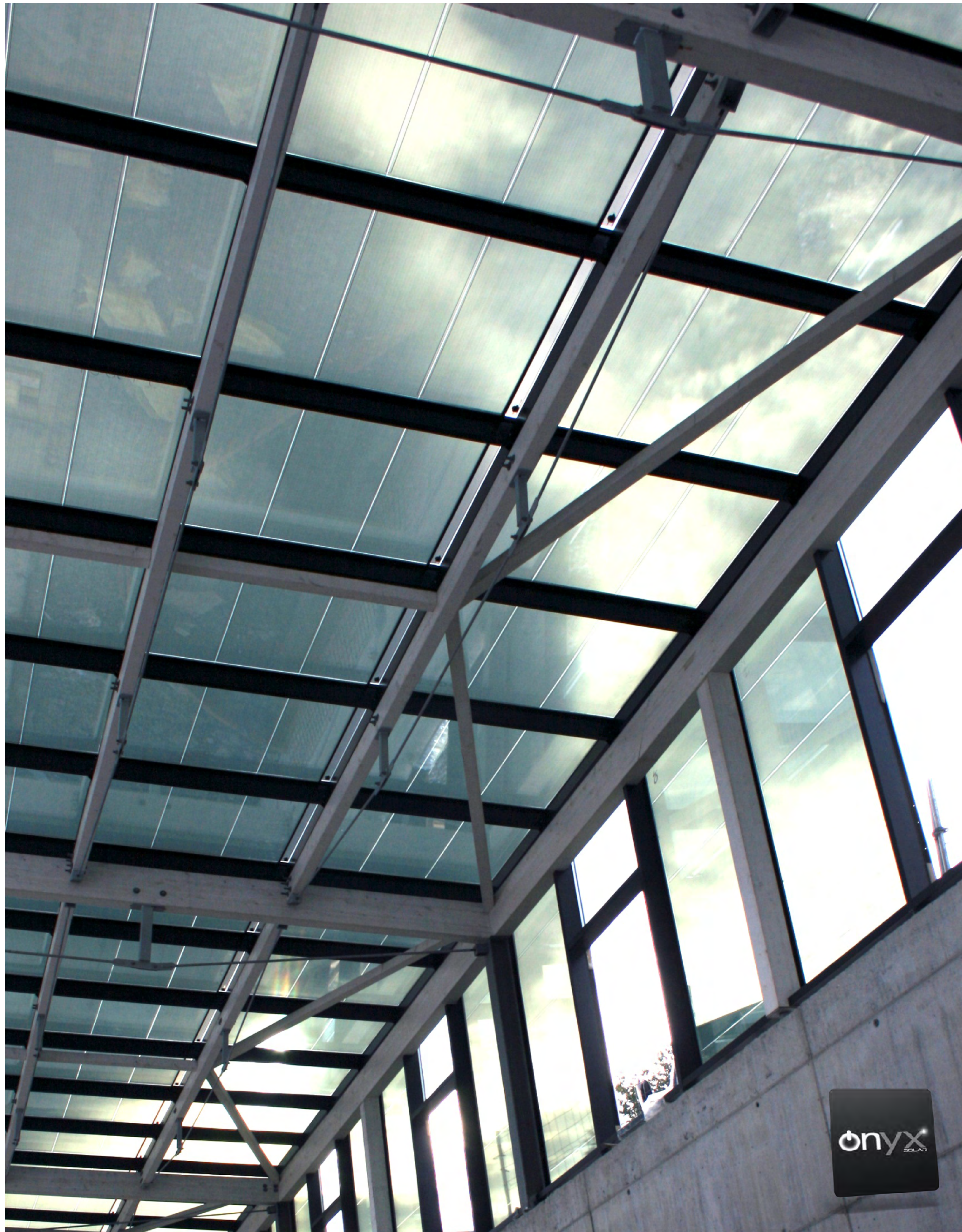
9-12. BIPV roof structure.
