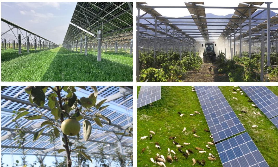
Figure 2: Some of the different agrivoltaics approaches. a) Top left: Large scale facility in China with moderate higher vertical clearance compared to GMPV, © Fraunhofer ISE; b) top right: Agrivoltaics in French viticulture; © Sun'Agri; c) bottom left: Apple farming in Germany, © Fraunhofer ISE; d) bottom right: Agrivoltaics with sheep grazing in USA, © Lindsay France, Cornell University. A more comprehensive classification of agrivoltaics can be found in Chapter 2.
