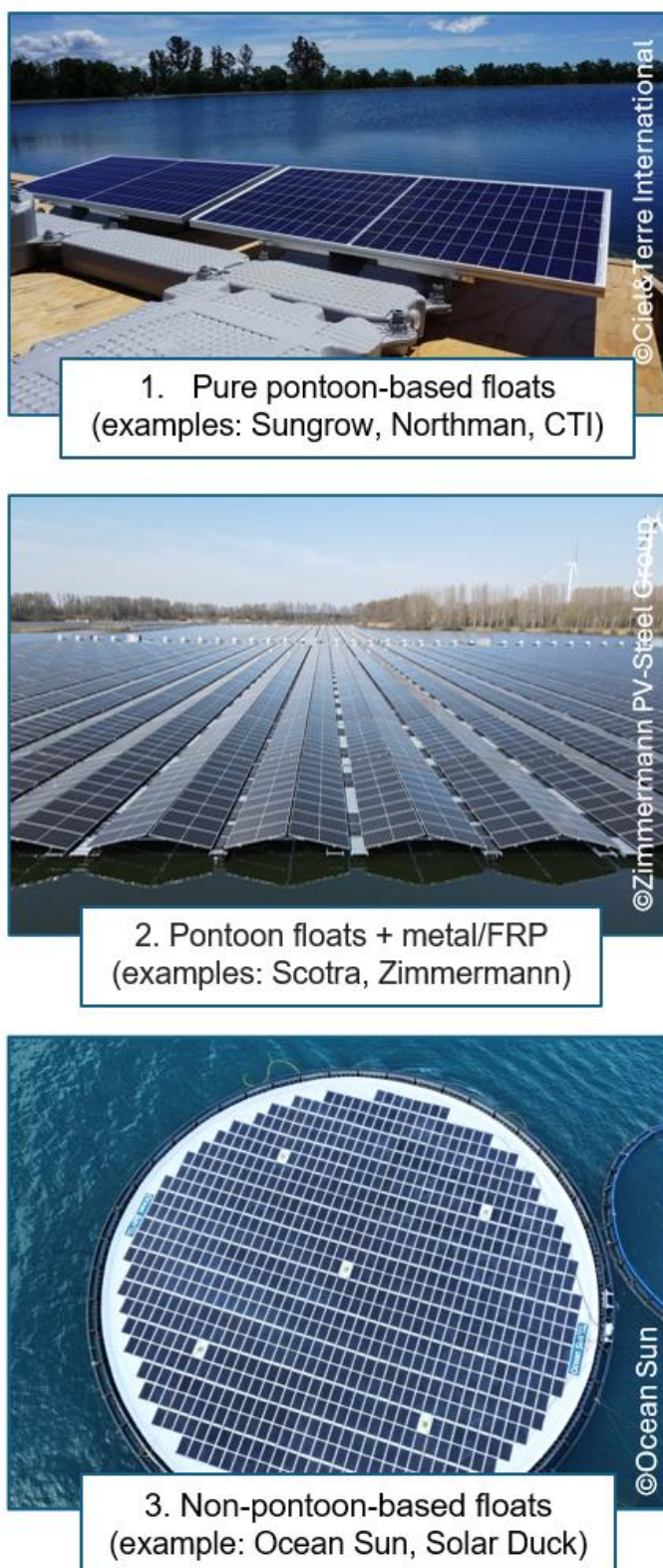
Figure 5. Categorization of FPV system based on float type. Illustration based on [3], [8], [121].
