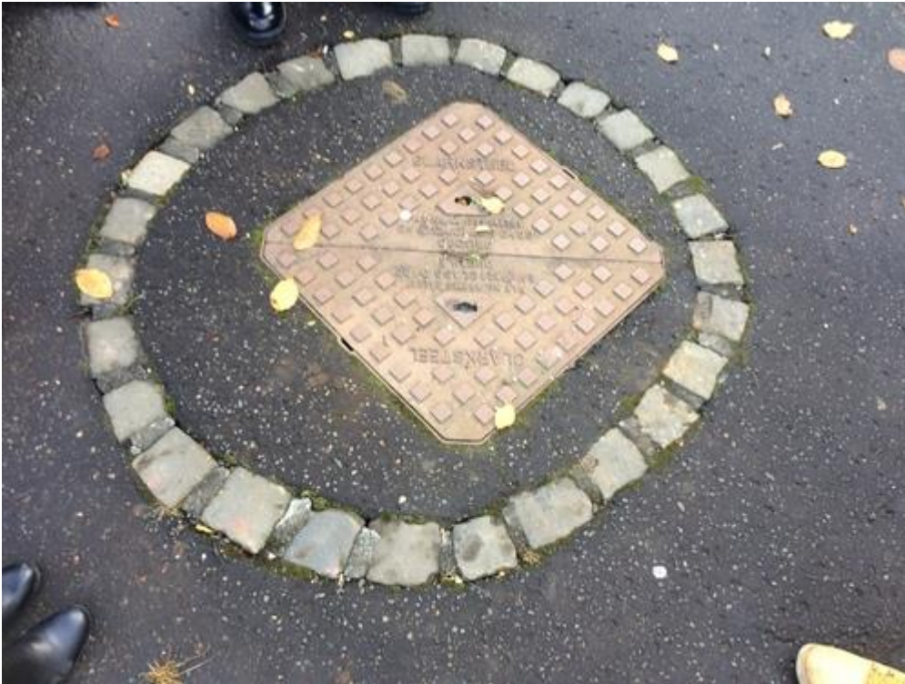
Figure 11: Puits de production.
