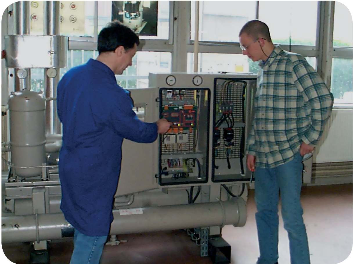
Technique maintenance. Source : www4b .
